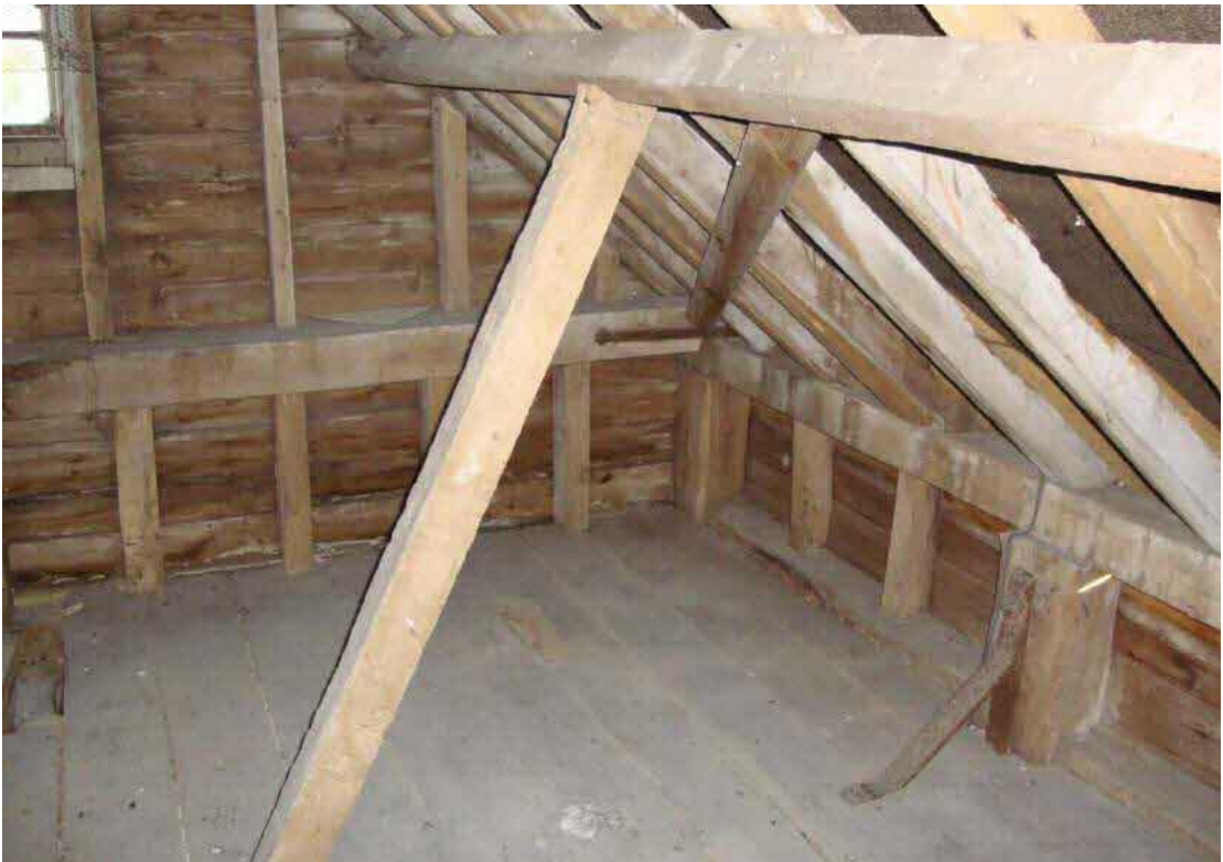
Fig.44 Wall and roof structure at east end of 'hoist loft'
