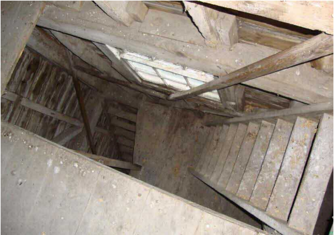
Fig.43 Ladder stairs that enabled internal movement between floors
