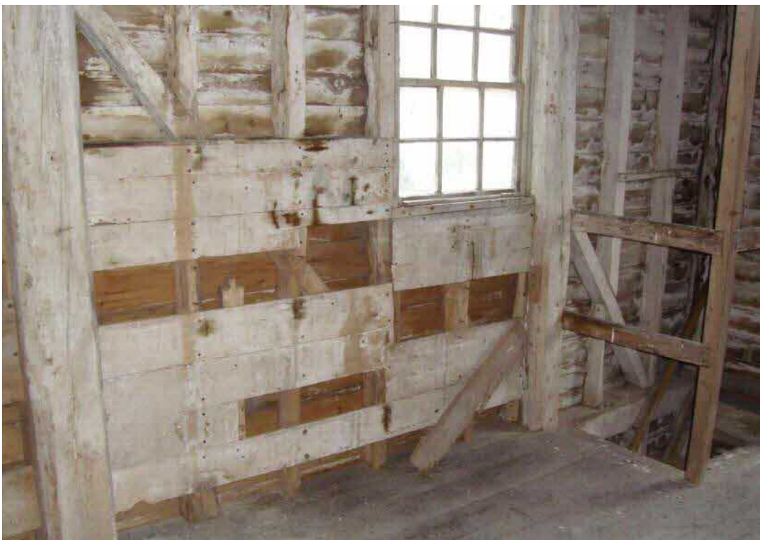
Fig.42 Walls lined with horizontal boarding on 'bin floor'
