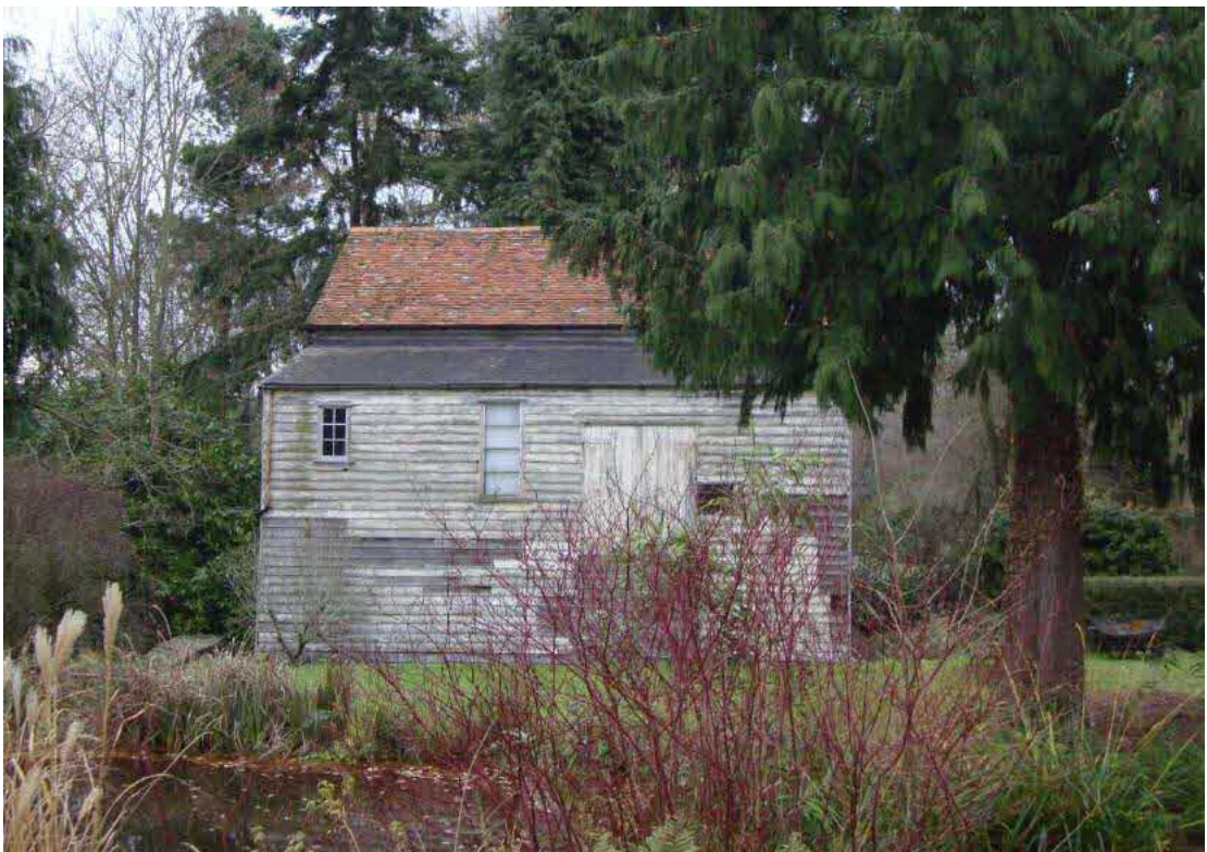
Fig.20 Lower Mill viewed from east bank of mill pond (8)
