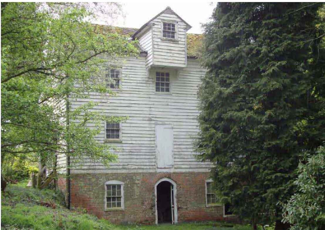
Fig.36 North façade of Shirburn 'Lower Mill' (built c.1800)
