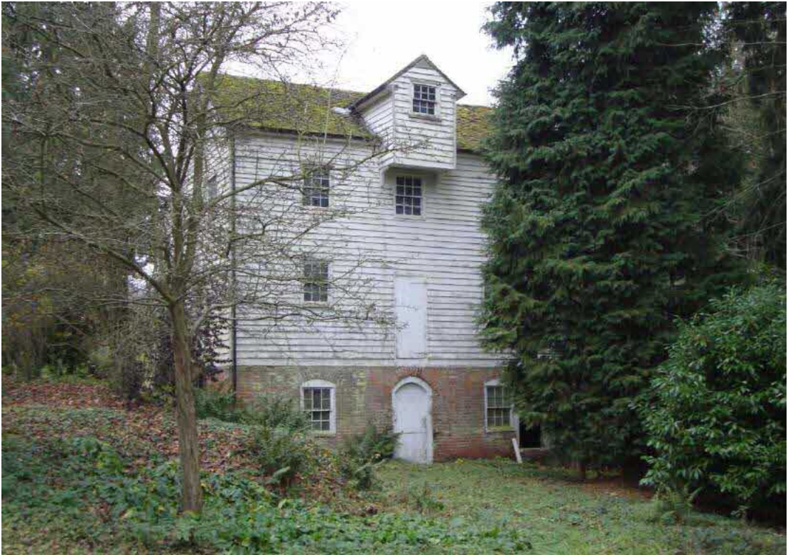
Fig.15 Lower Mill viewed from internal access track to north (3)
