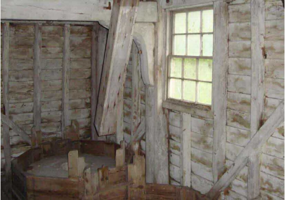
Fig.40 Timber-framed structure and internal finishes on 'stone floor'
