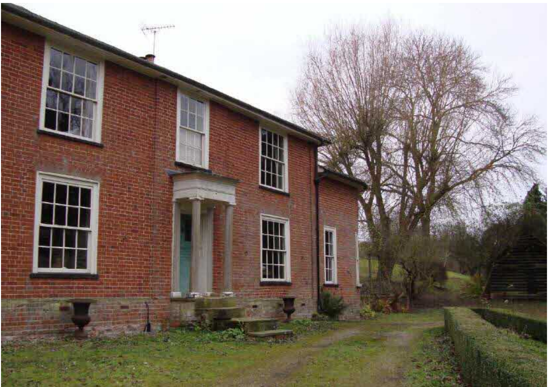
Fig.16 View south across front of Mill House (4)
