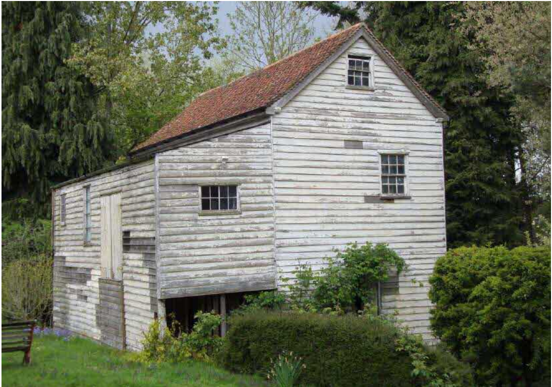
Fig.46 Shirburn Mill as enlarged in the early twentieth century
