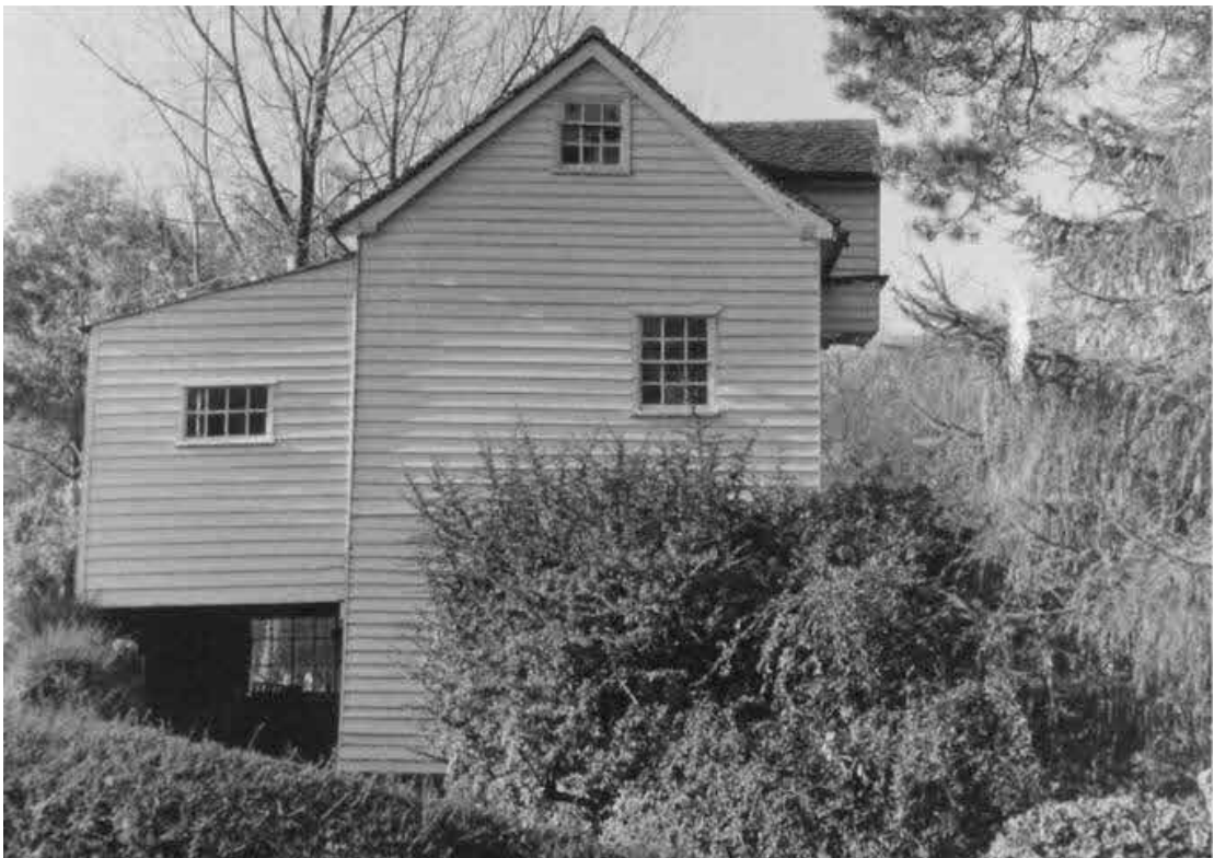
Fig.11 Side (east) elevation of Shirburn 'Lower' Mill, 1966
