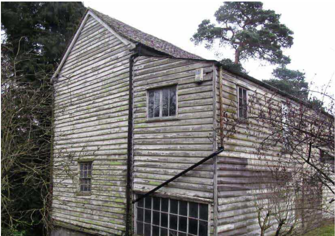
Fig.49 Shirburn Mill from south-west, c. 1990
