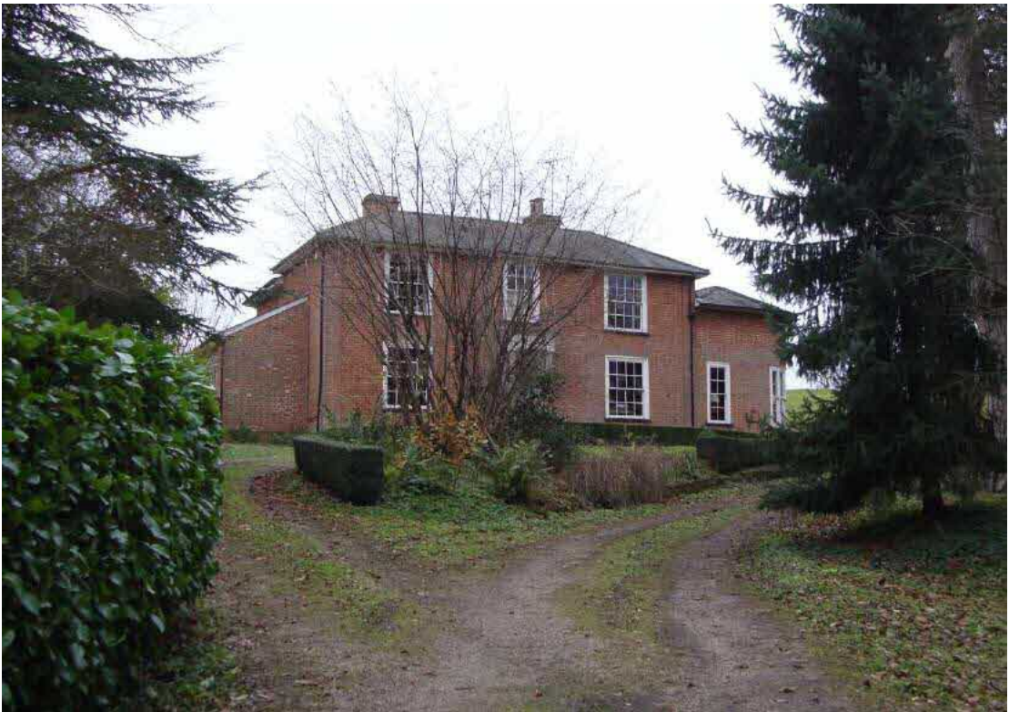
Fig. 14 Mill House viewed from internal access track to north (2)
