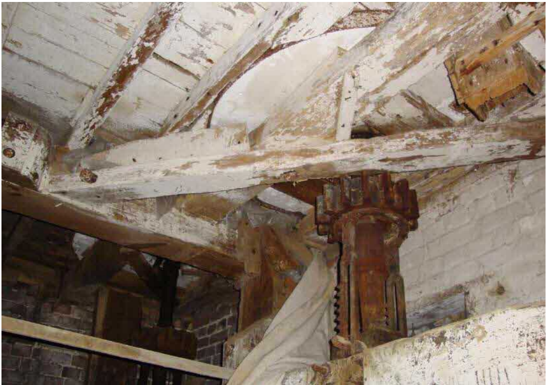
Fig.38 Two stone nuts and shafts attached to millstones above
