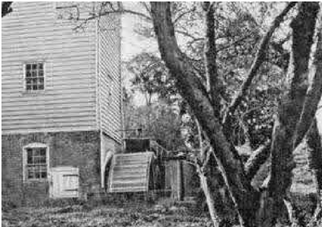
Fig.37 Exterior overshot waterwheel at Shirburn Mill, c.1910
