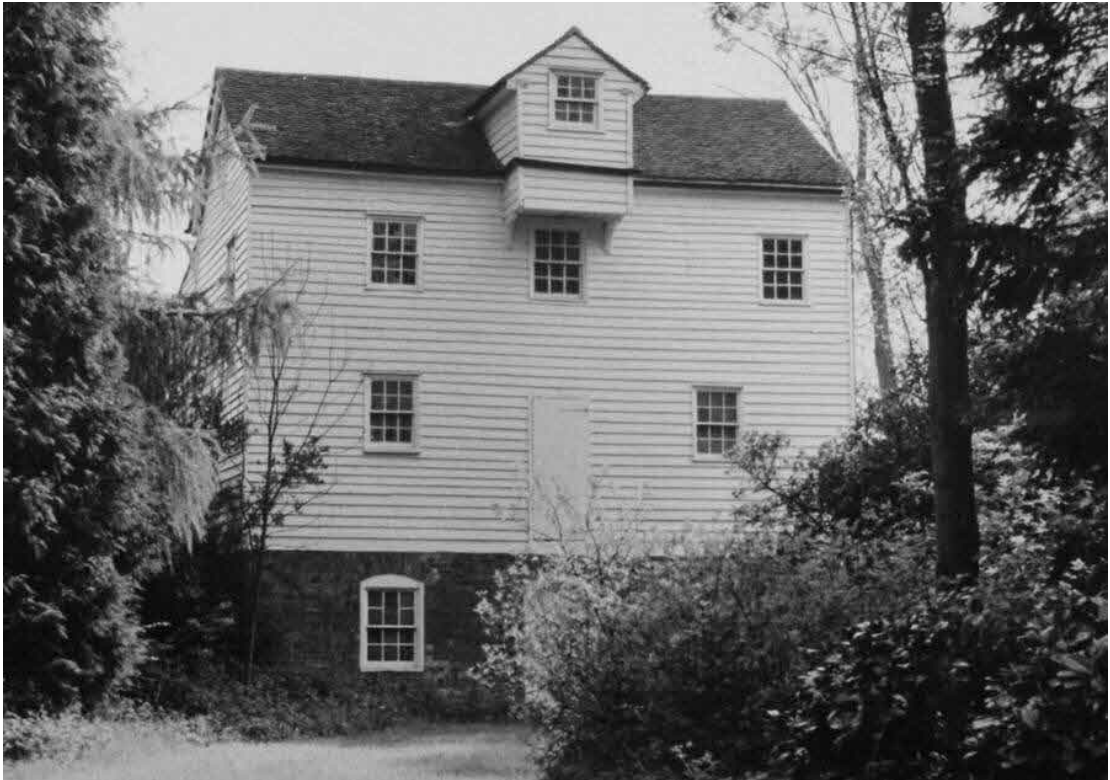
Fig.9 Principal (north) elevation of Shirburn 'Lower' Mill, 1966
