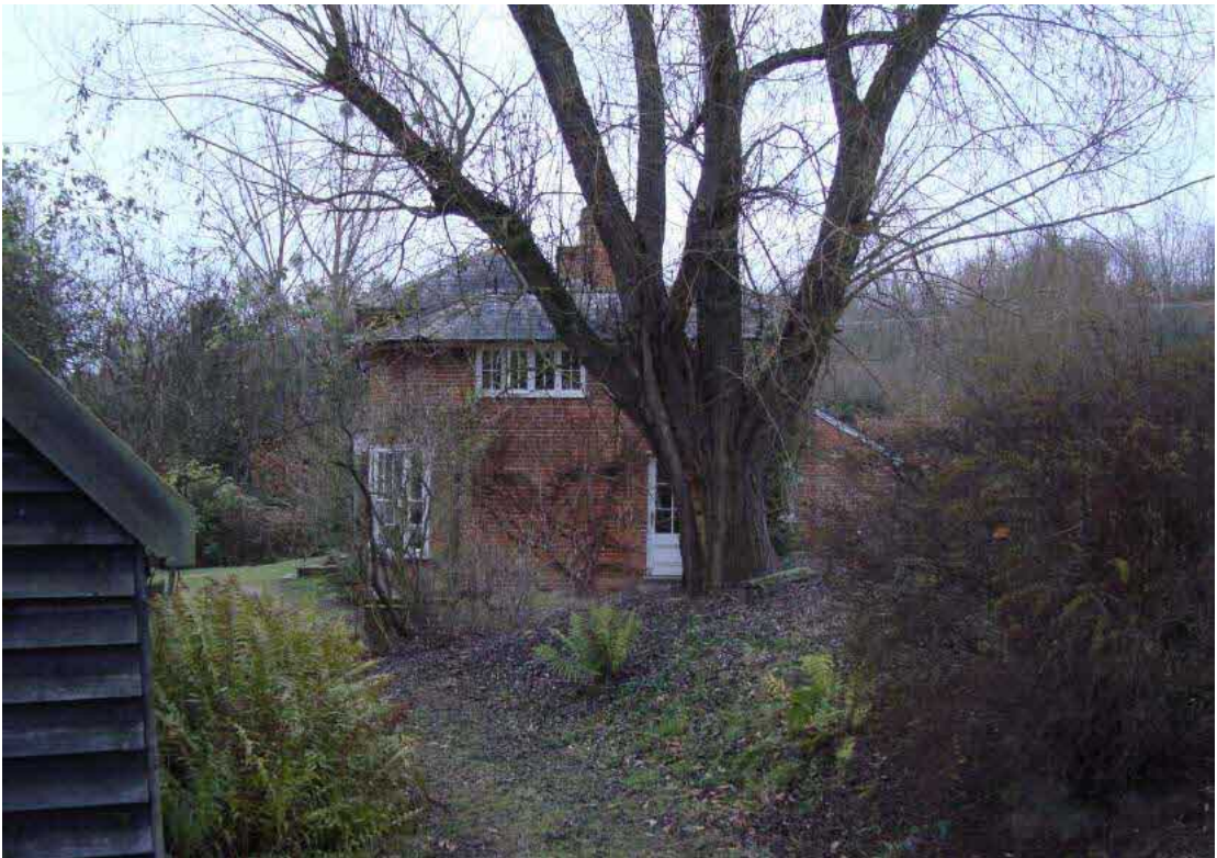
Fig.18 Mill House viewed from internal access track to south (6)
