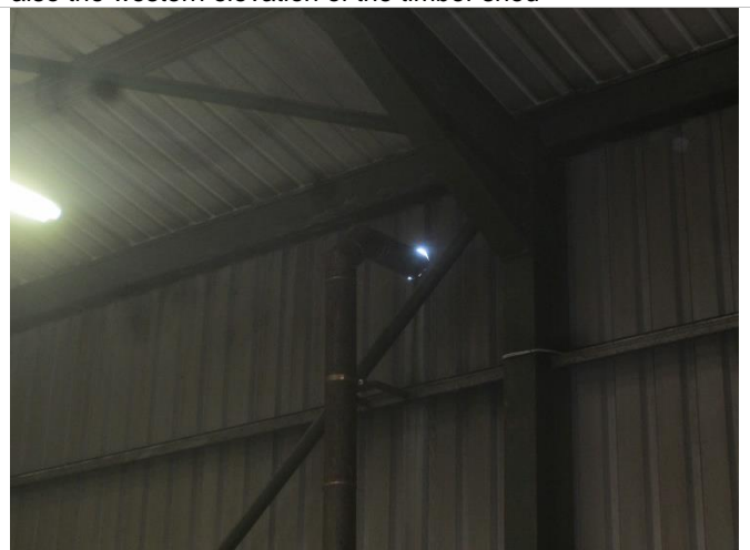
Photo 18: Interior of Building 1
