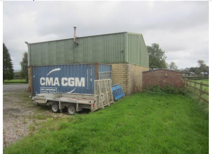
Photo 16: Western and southern elevations of Building 1 and also the western elevation of the timber shed
