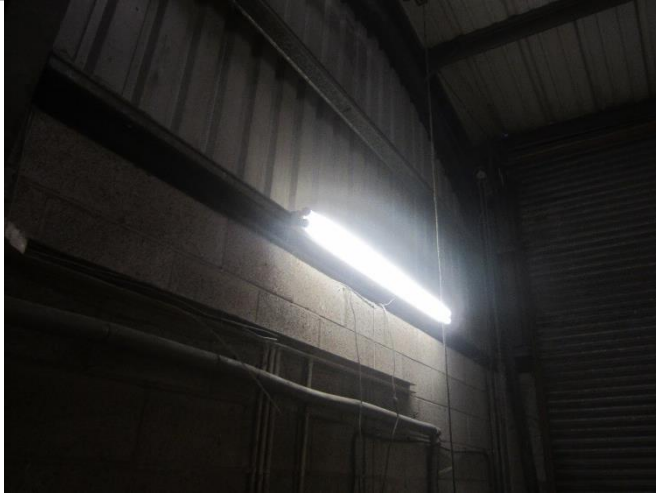
Photo 19: Interior of Building 1
