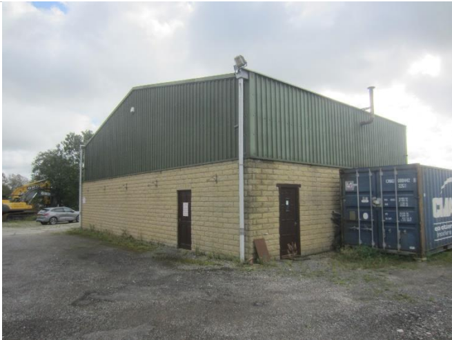
Photo 15: Northern and eastern elevations of Building 1: Workshop
