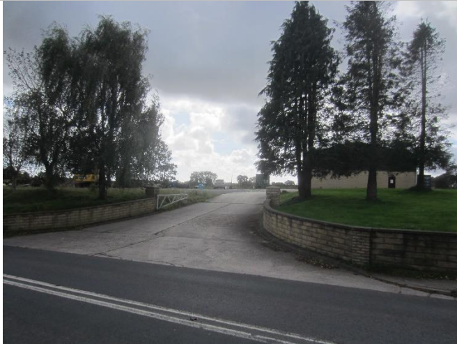
Photo 1: Site entrance off Preston Road with brick walls
