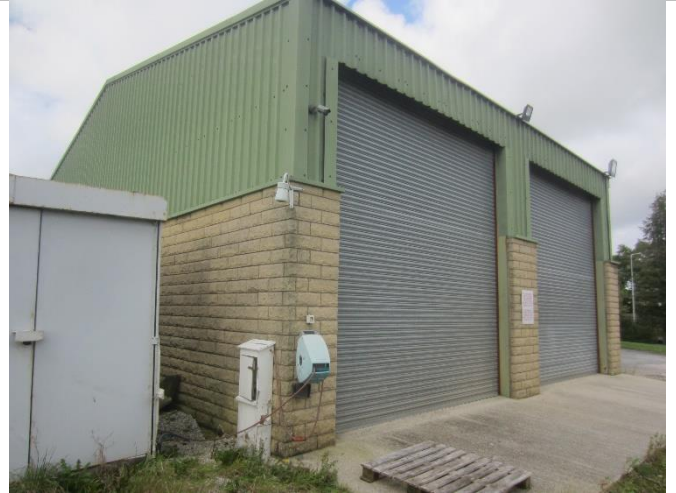
Photo 14: Southern and western elevations of Building 1: Workshop
