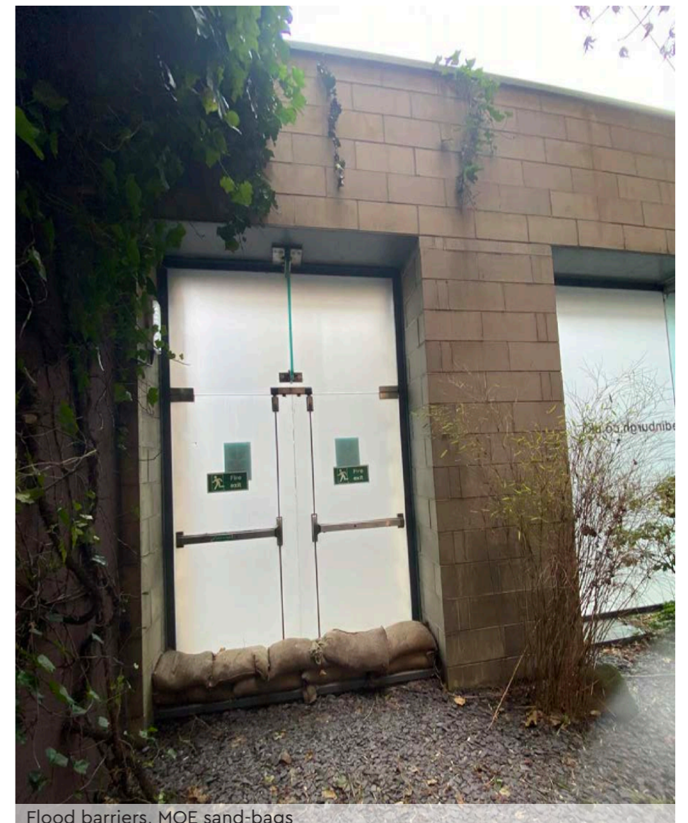
Flood barriers on lower-ground floor
