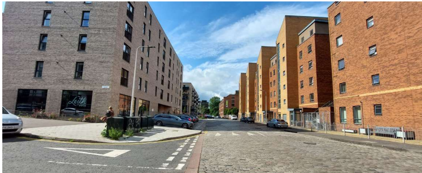
B / View looking South along Salamander Place
