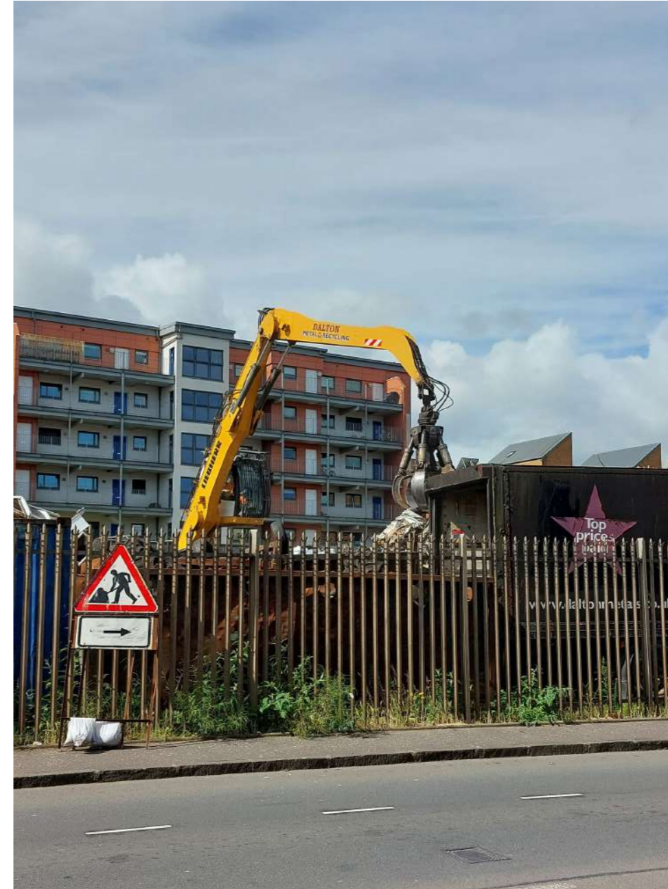
C / View of the Site Looking South-West Showing the Machinery.
