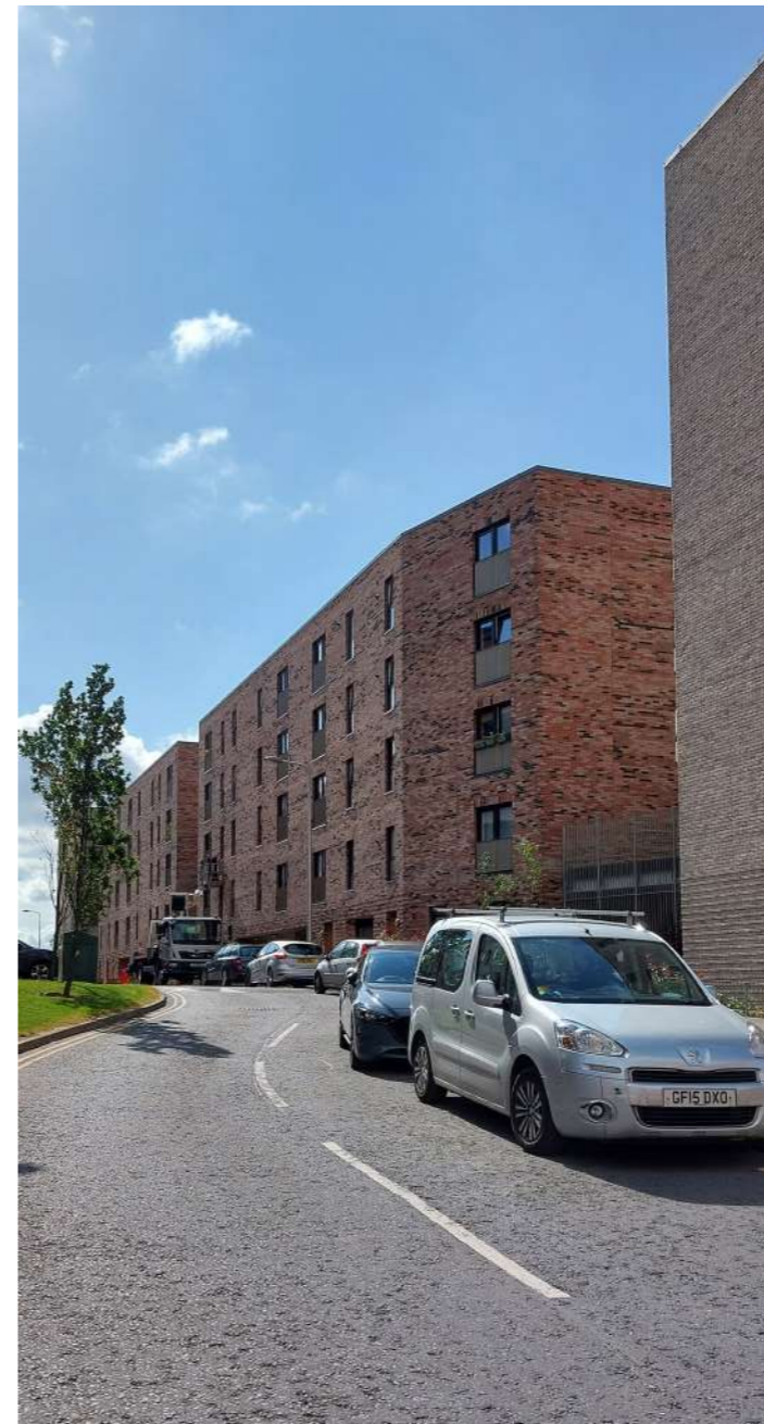
C / View looking East along Sailmaker Road
