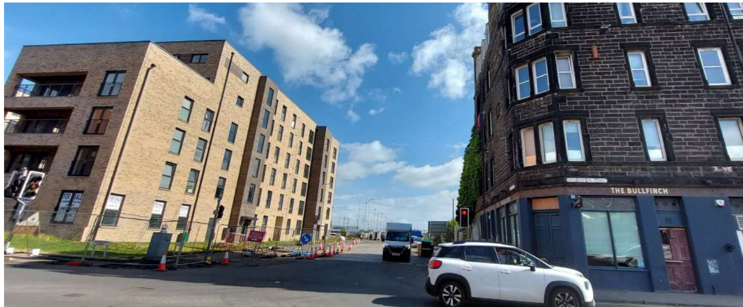
A / View from the corner of the site looking North down Bath Road to Forth Ports
