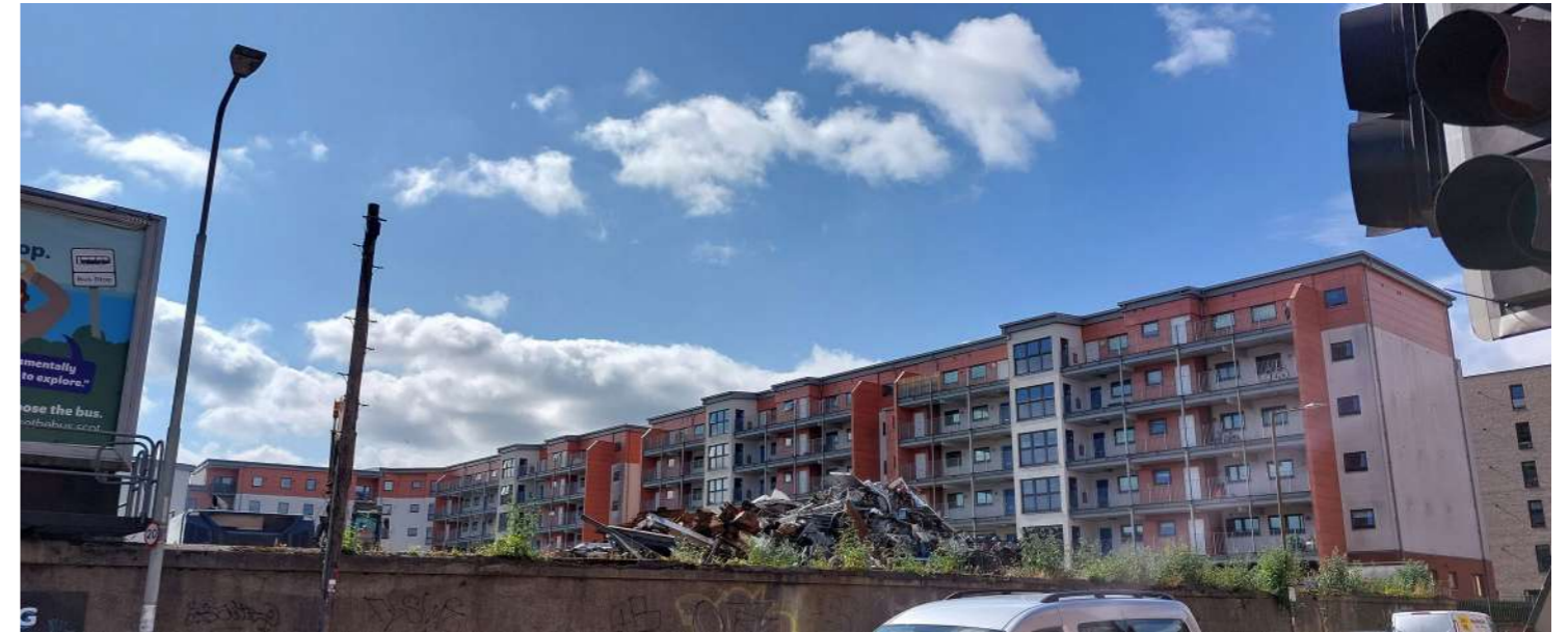
B / View of the Site Looking South-East
