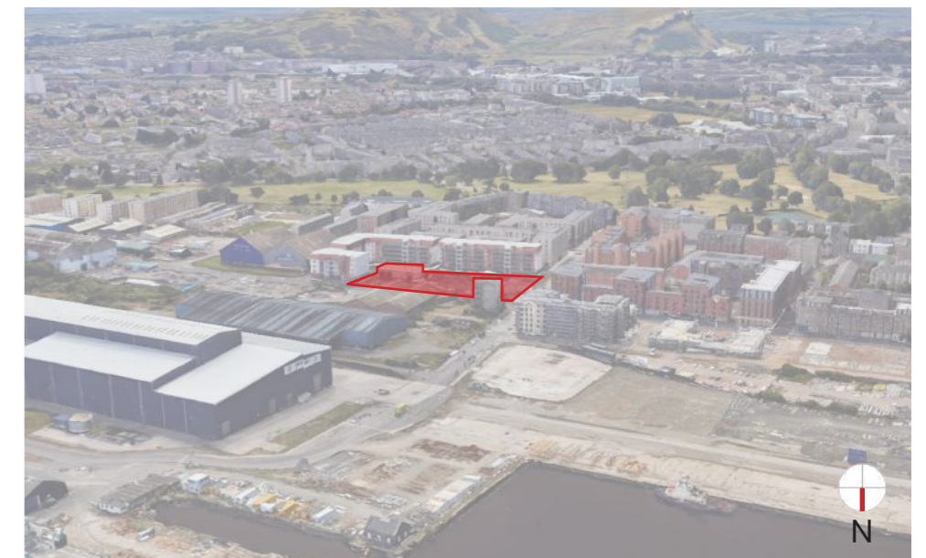
B / View of the Site looking South towards Arthur's Seat
