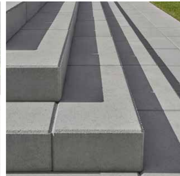
Bespoke concrete stair at the entrance area
