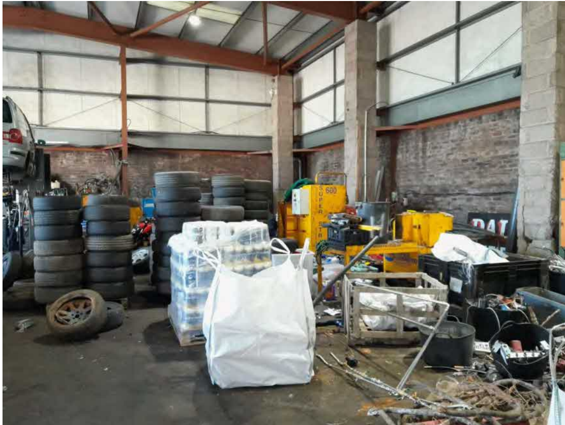
Plate 3: Photo facing the south-east corner of the building, containing stacks of tires and various car equipment/parts.
