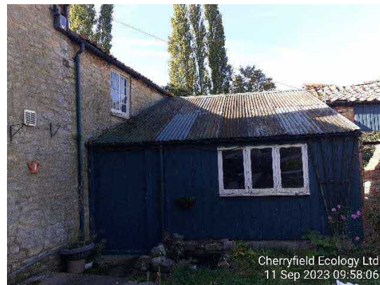
Figure 5- Wooden paneled building joined to the main house.
