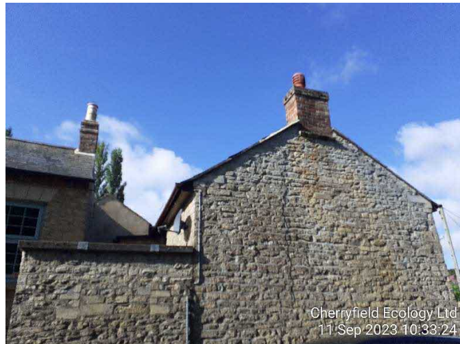
Figure 3- Main house with external walls and windows (B1).
