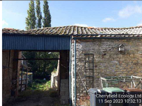
Figure 8- Building (B1b) with clay tile roof.
