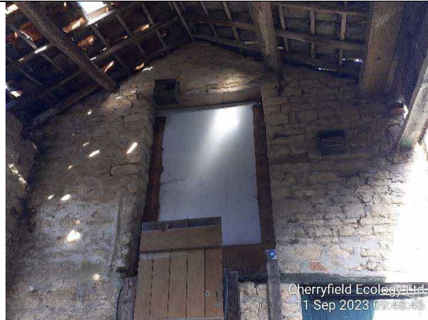
Figure 10- Interior wall of building with door.
