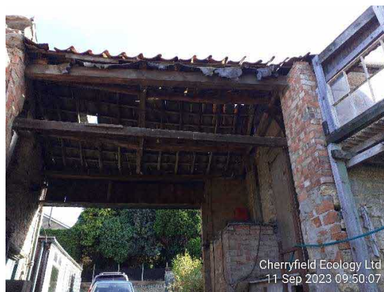
Figure 12- Underside of roof.
