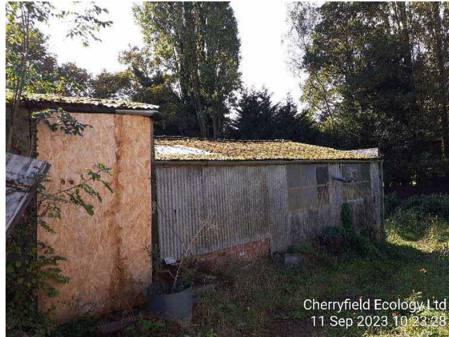
Figure 13-Metal sheet building joined to the main house.
