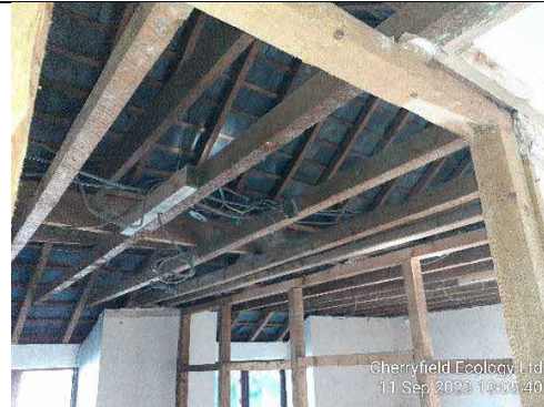
Figure 4- Exposed joists and rafters in second storey of the house.
