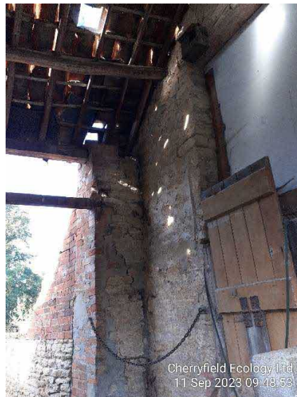
Figure 11- Internal brickwork of building.
