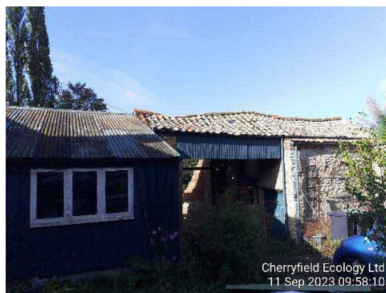
Figure 7- Pitched roof joining the buildings.
