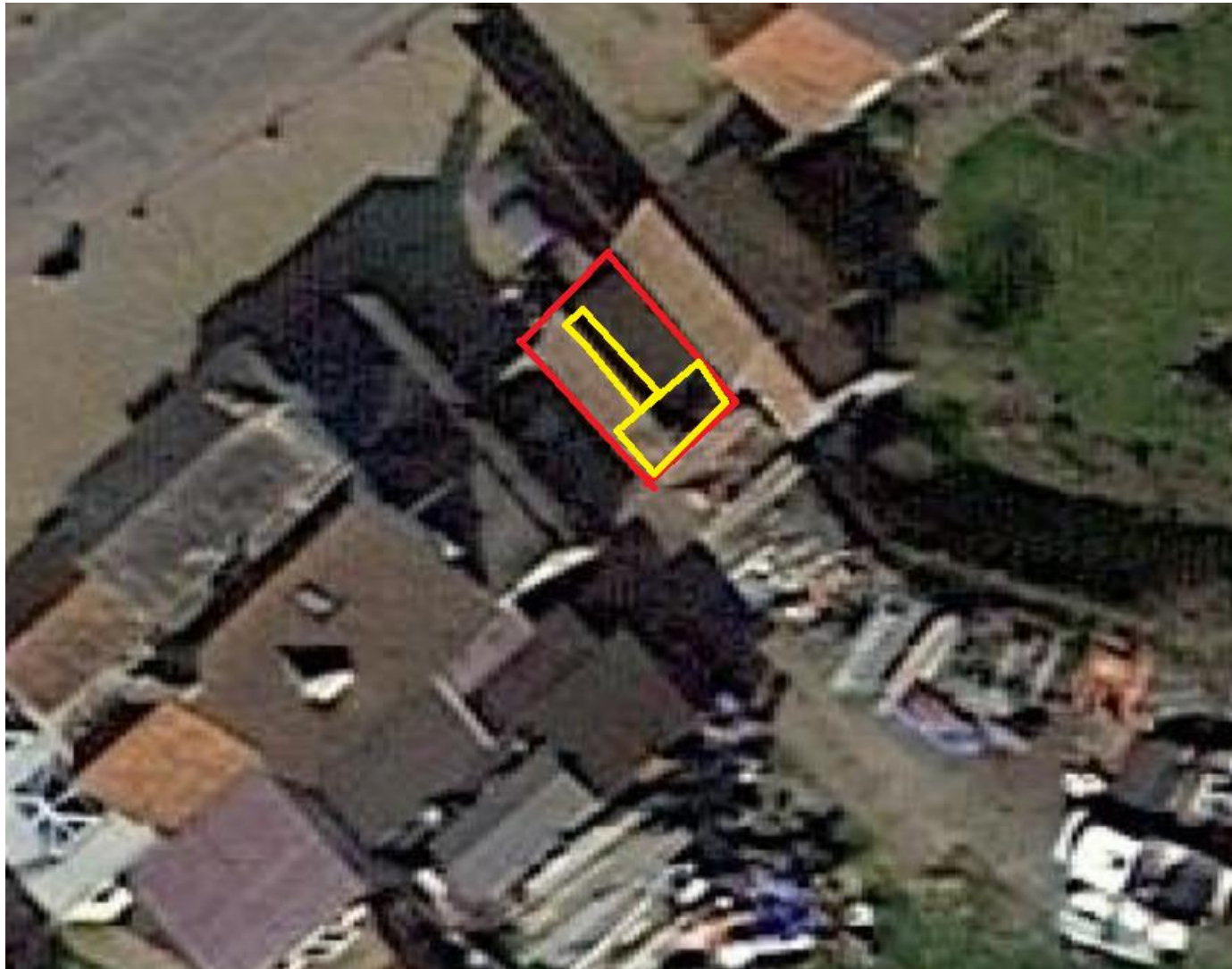
Building surveyed – Red outline boundary, Areas of neglect and damage giving lots of exposure.
