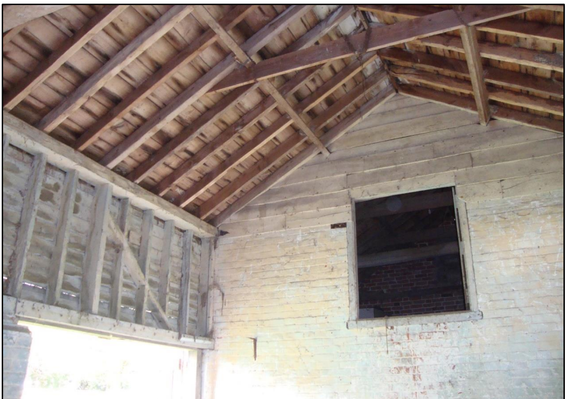
Fig.46 Interior of former coach-house
