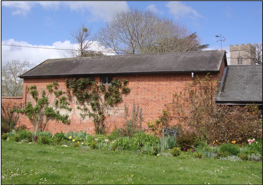
Fig.23 Rear of mid-nineteenth century building
