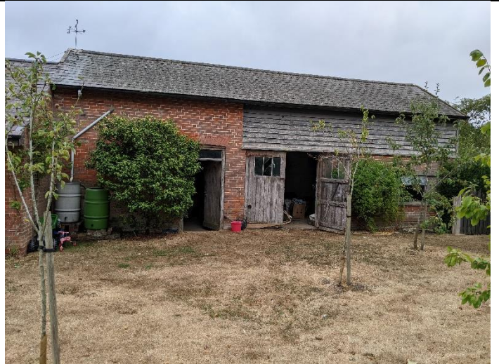
Photo 2 Northwest elevation of existing barn B2
