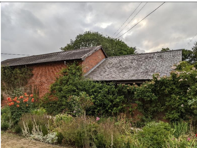
Photo 5 Southwest elevation of garage proposed for demolition B3
