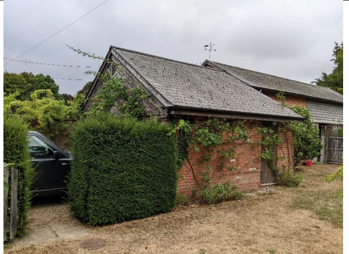
Photo 4 Northwest elevation of garage proposed for demolition B3
