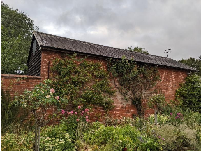
Photo 3 Southwest elevation of existing barn B2
