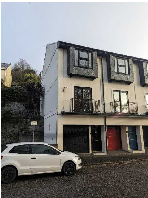
Photo 1. Showing the front of the house from the east
