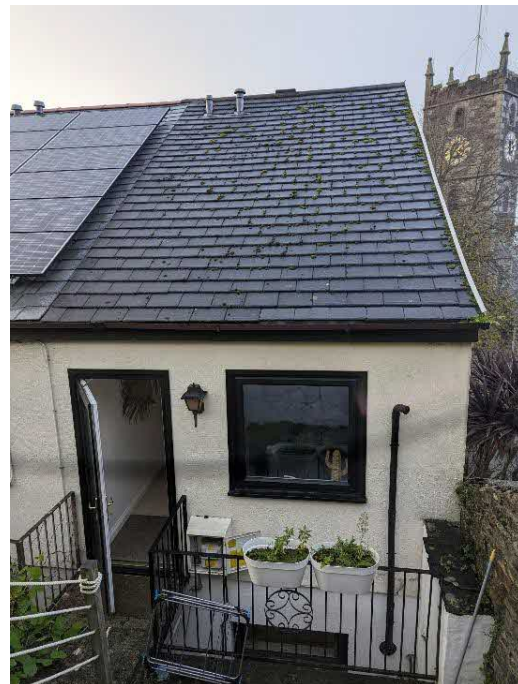
Photo 2. Showing the rear of the house from the west
