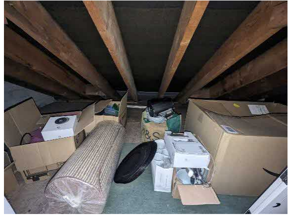
Photo 4. Showing the remaining area of roof void to the front
