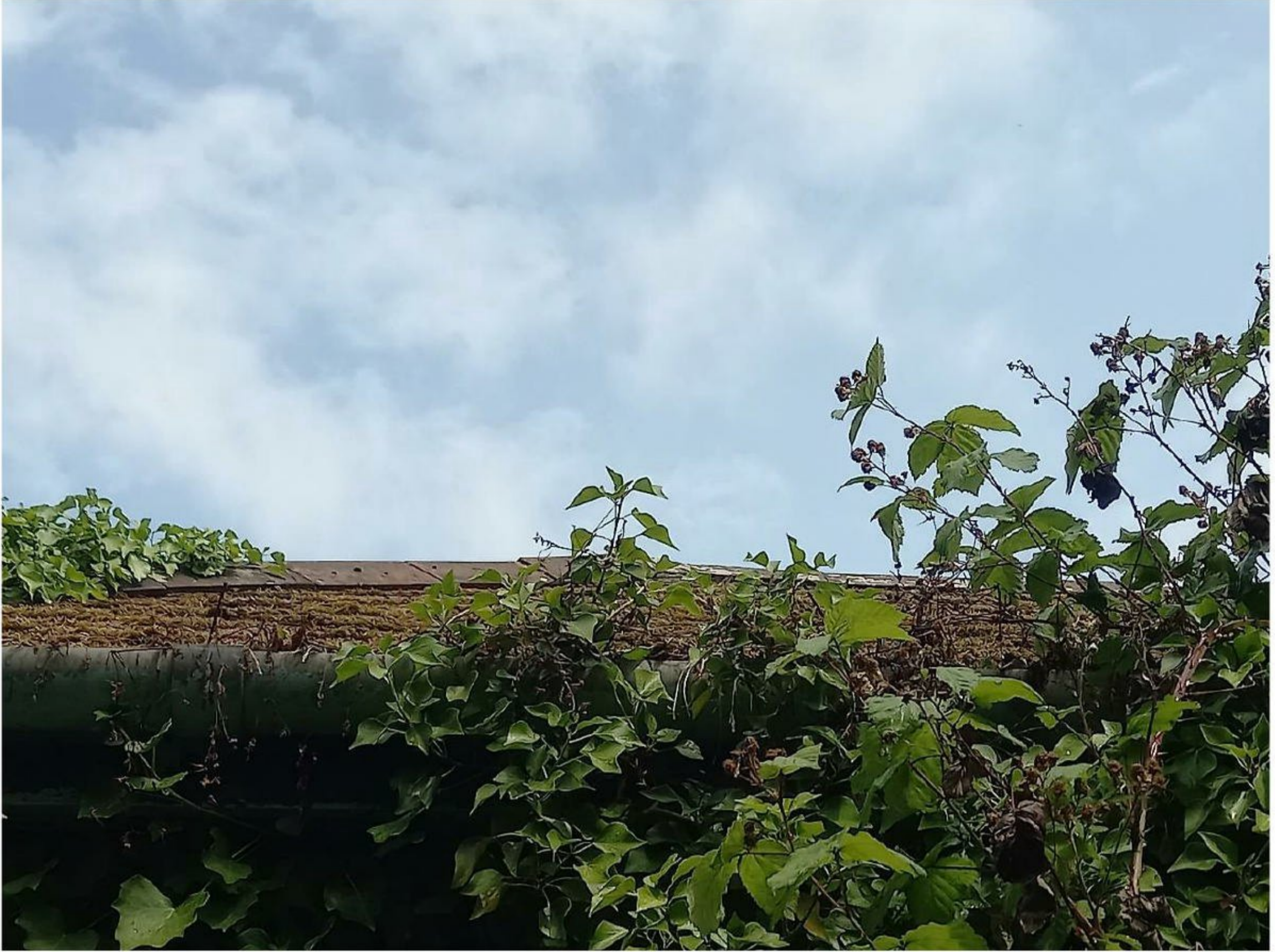
Plate 15 – Roof of building 4.
