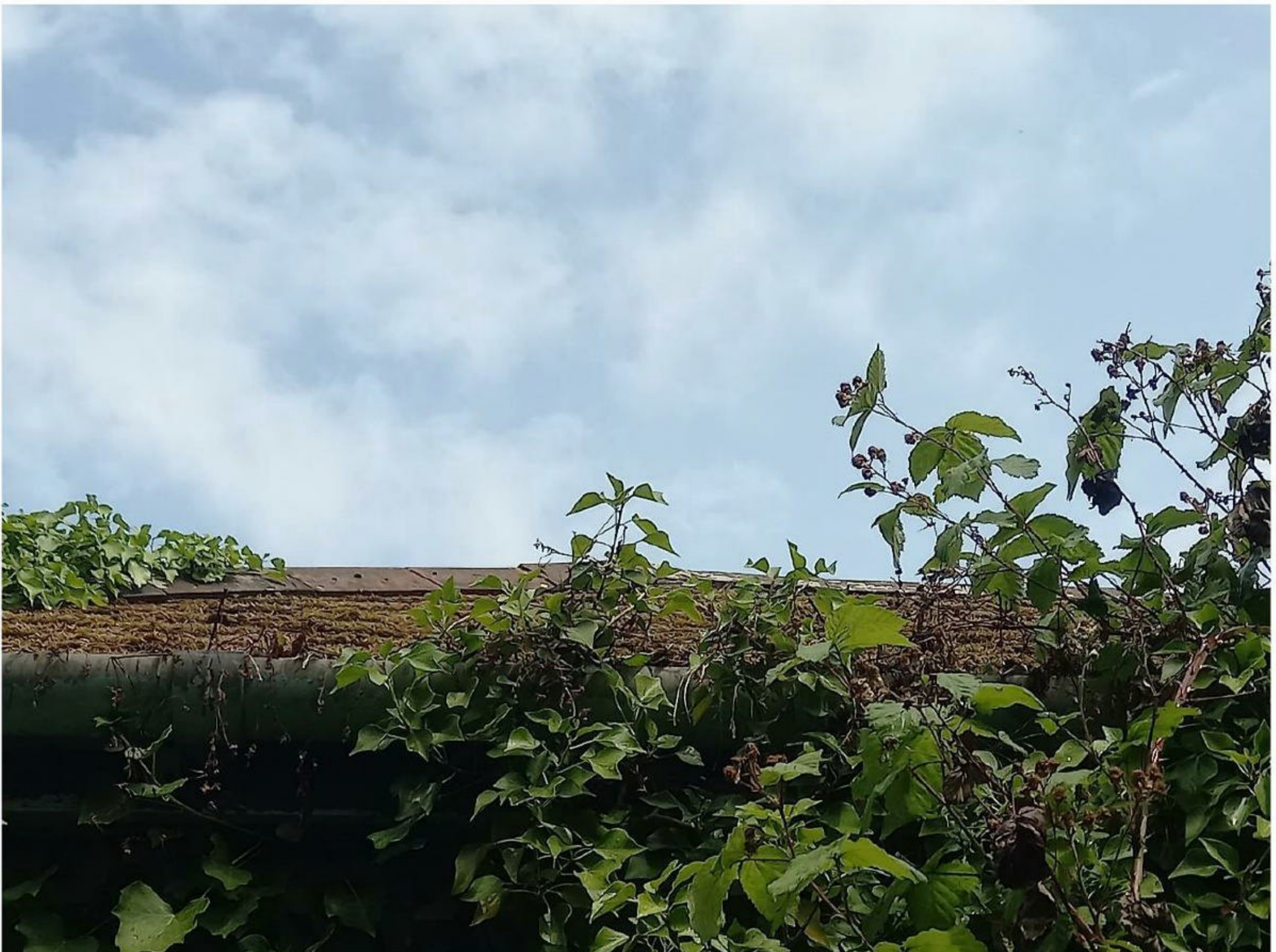
Plate 16 – Roof of building 4.
