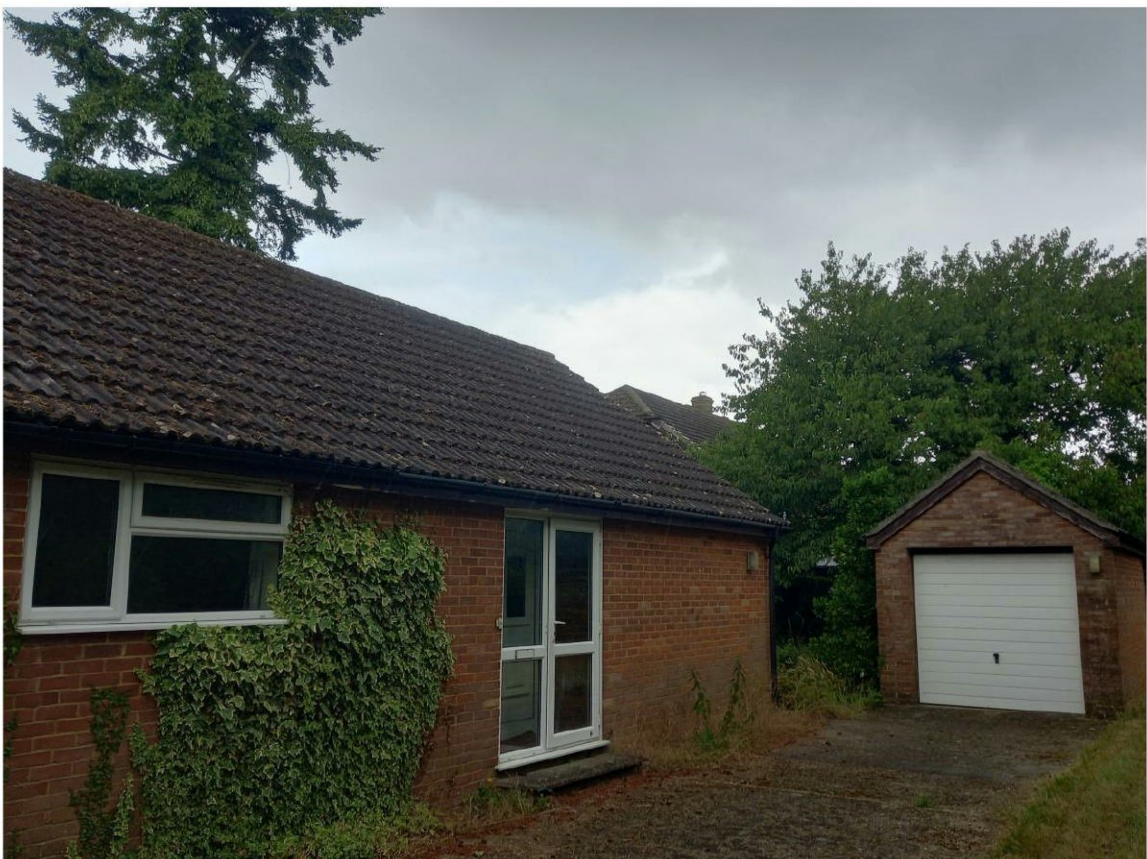
Plate 6 – Eastern aspect of building 1, building 2 also seen.
