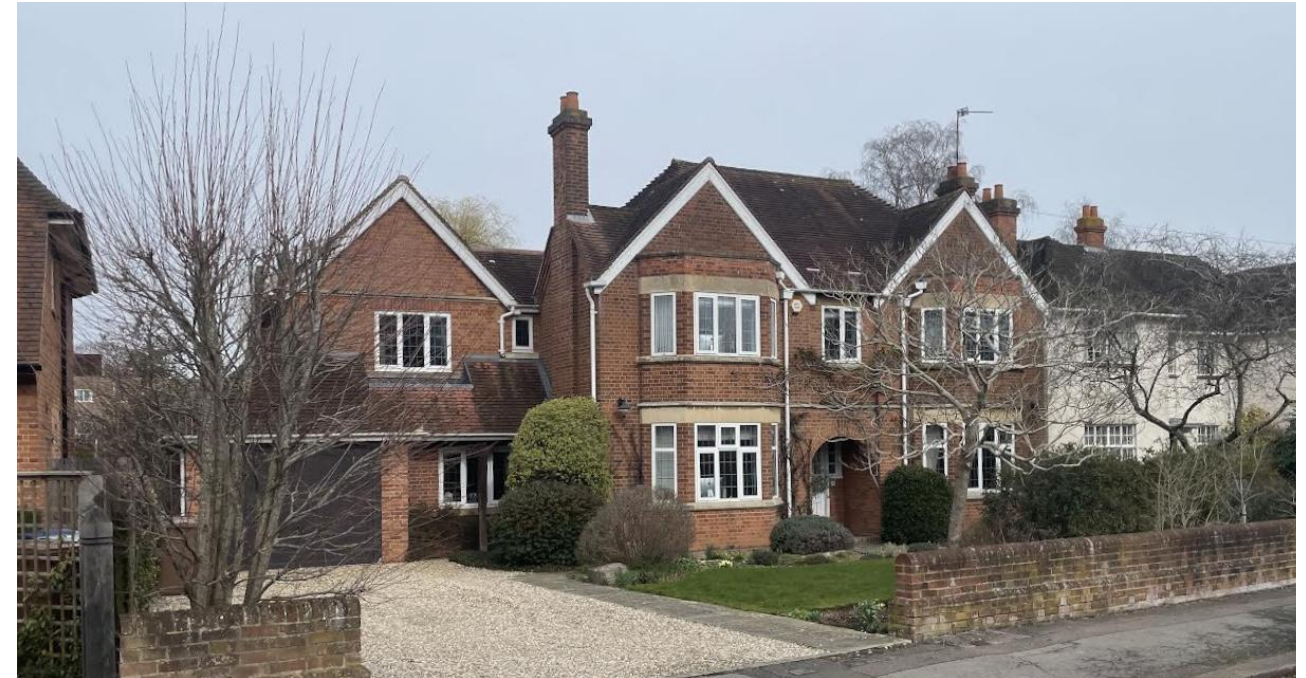
Photo taken of no.11 from Belbroughton Road (No.9 on the left. No.13 on the right )
