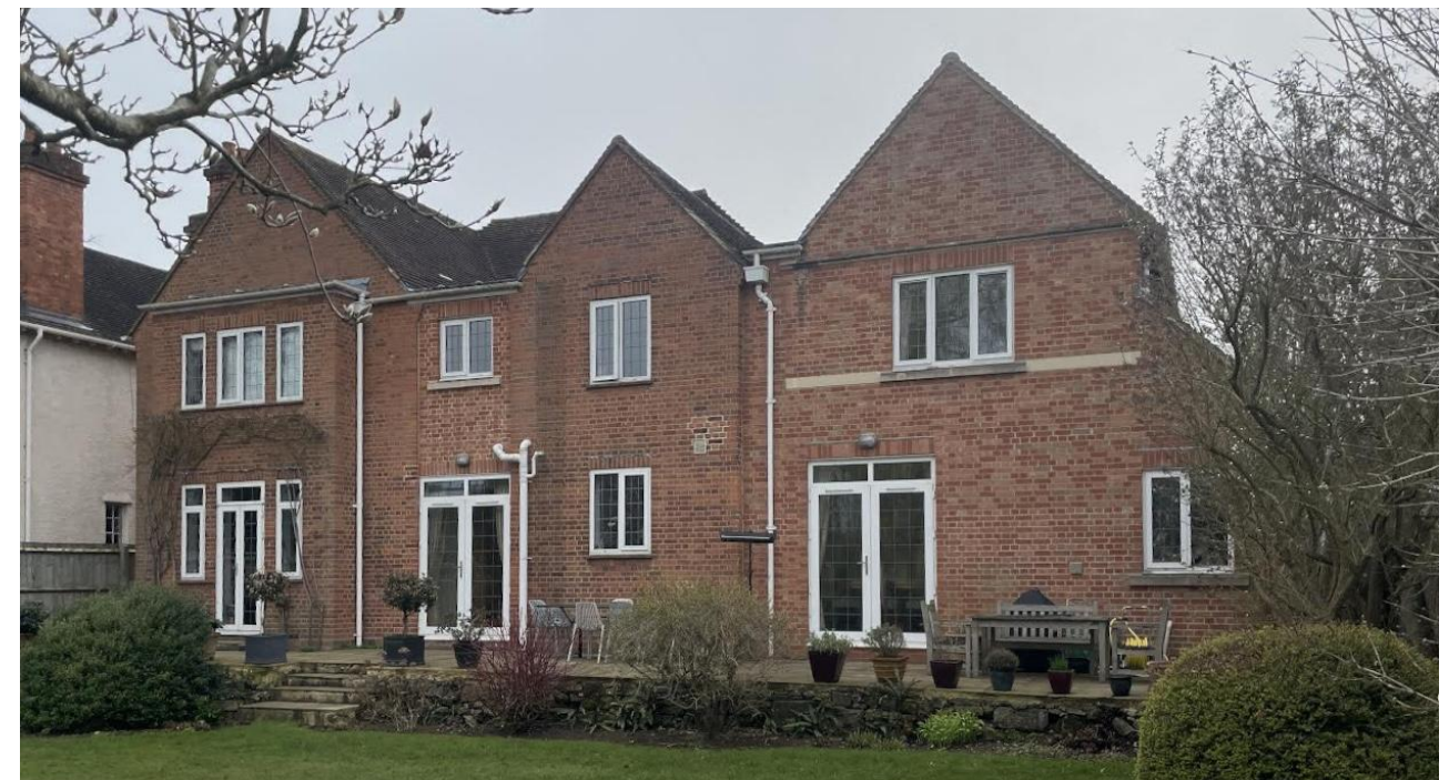
Photo taken of no.11 from the rear garden
