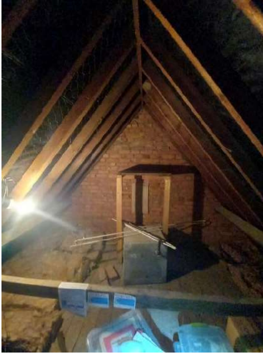
Photo 5: North end of principal loft with ventilation slit in gable wall boarded over internally
