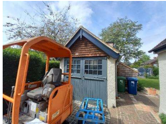
Photo 4: South elevations of garage/outbuilding
