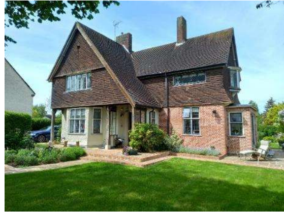
Photo 2: South and east elevations
