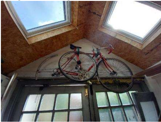
Photo 11: Internal area of garage (south end)
