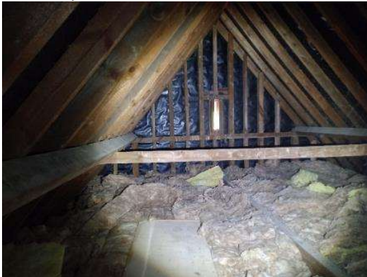
Photo 7: South end of principal loft with metal grille over ventilation slot
