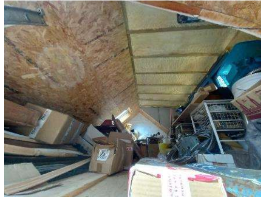
Photo 10: Internal 'loft' area of garage (south end)
