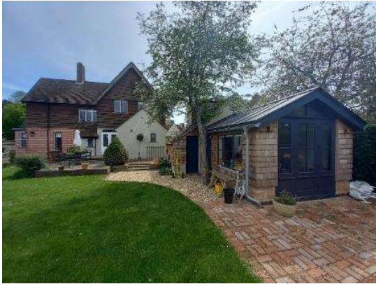
Photo 9: North and east elevations of garage/outbuilding
