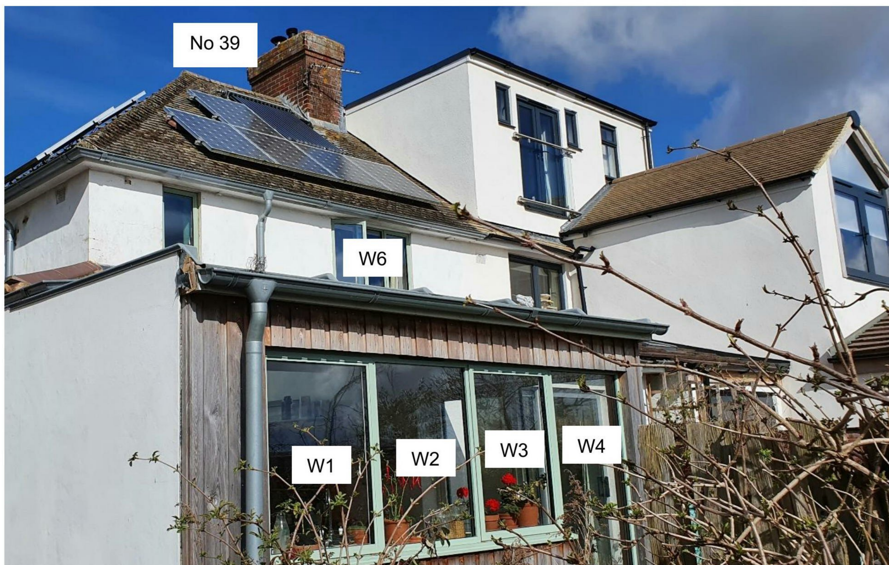
Figure 2 Photograph (taken during site visit) showing the analysed kitchen and bedroom windows at 39 Meadow Prospect, labelled W1 to W4 and W6, respectively.
