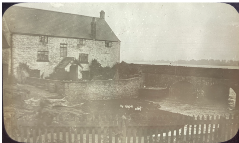
Drakes House, c. 1900, showing external limewash, blocked window and chimney (removed in 1960's). Note also the external quayside wall, parts of which survive.
