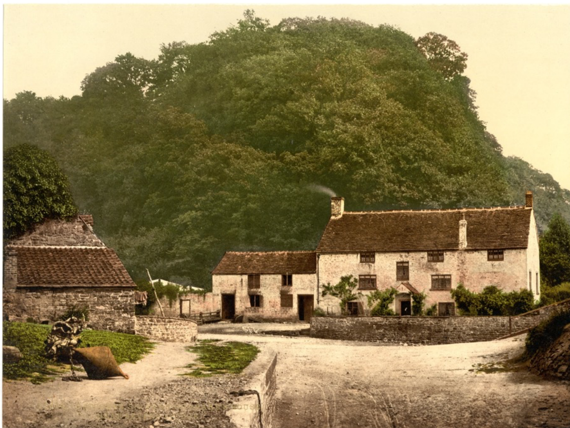
Drakes House – coloured photograph, now in Library of Congress, taken around 1890
