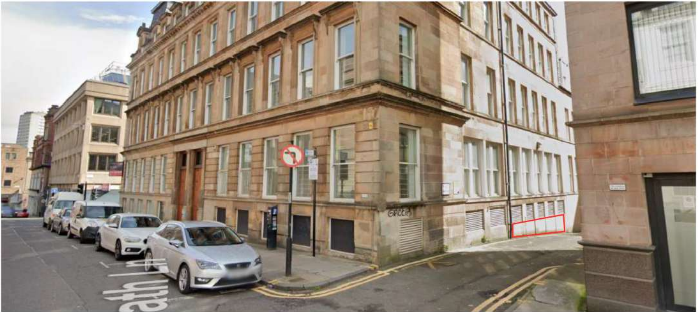
Figure 2 shows the location of this as viewed from Wellington Street. The additional louvres are designed to sit within the existing pilasters, with the existing openings cut down to provide the additional ventilation space required. The client is proposing to paint these louvres to match the colour of the surrounding stone, as has been done with those that are existing in order to reduce their visual impact.
