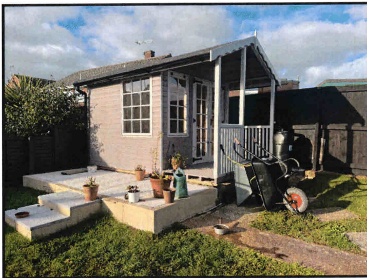
South and East Elevations
