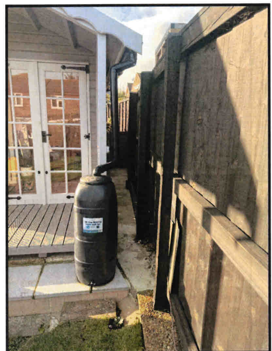
North Elevation Adjacent to Footpath Starting at Ground Level
