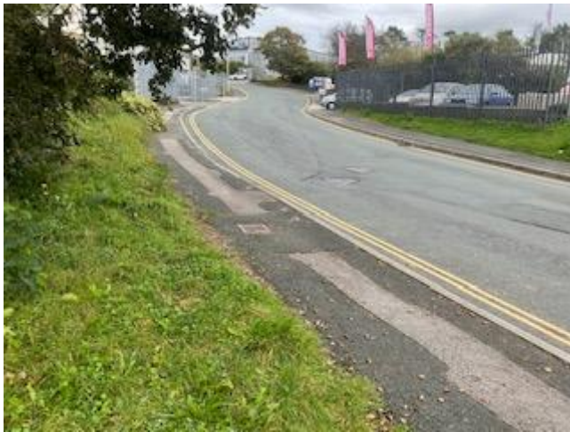
Figure 1: Aligned tree-line could restrict visibility at access.
