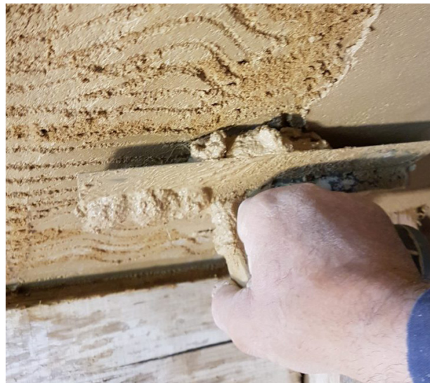
Lime plaster top coat
