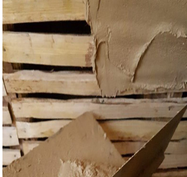
Lime plaster scratch coat
