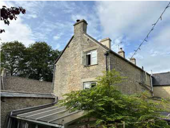
3: East gable end.
