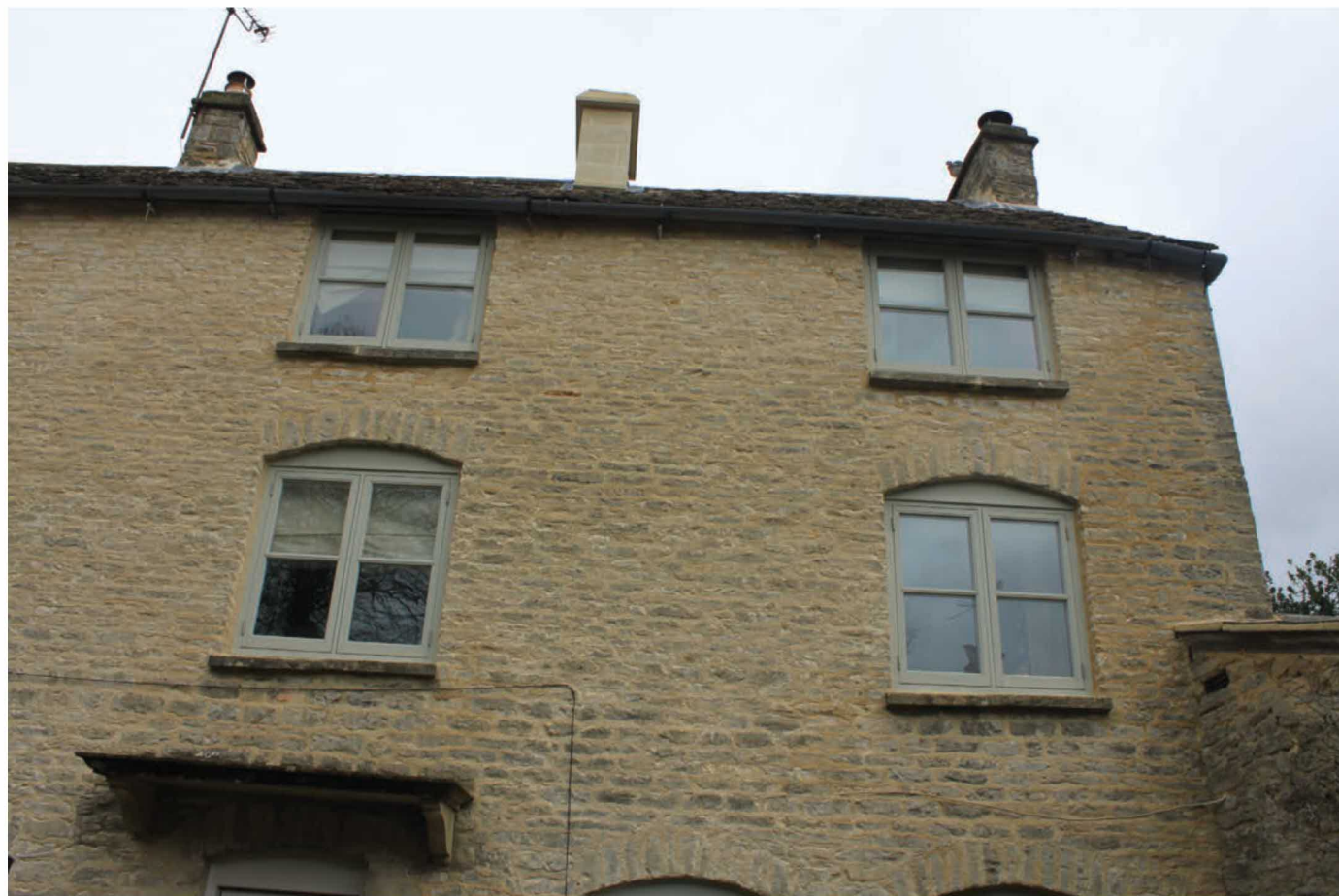
Front elevation showing the upper floors.
