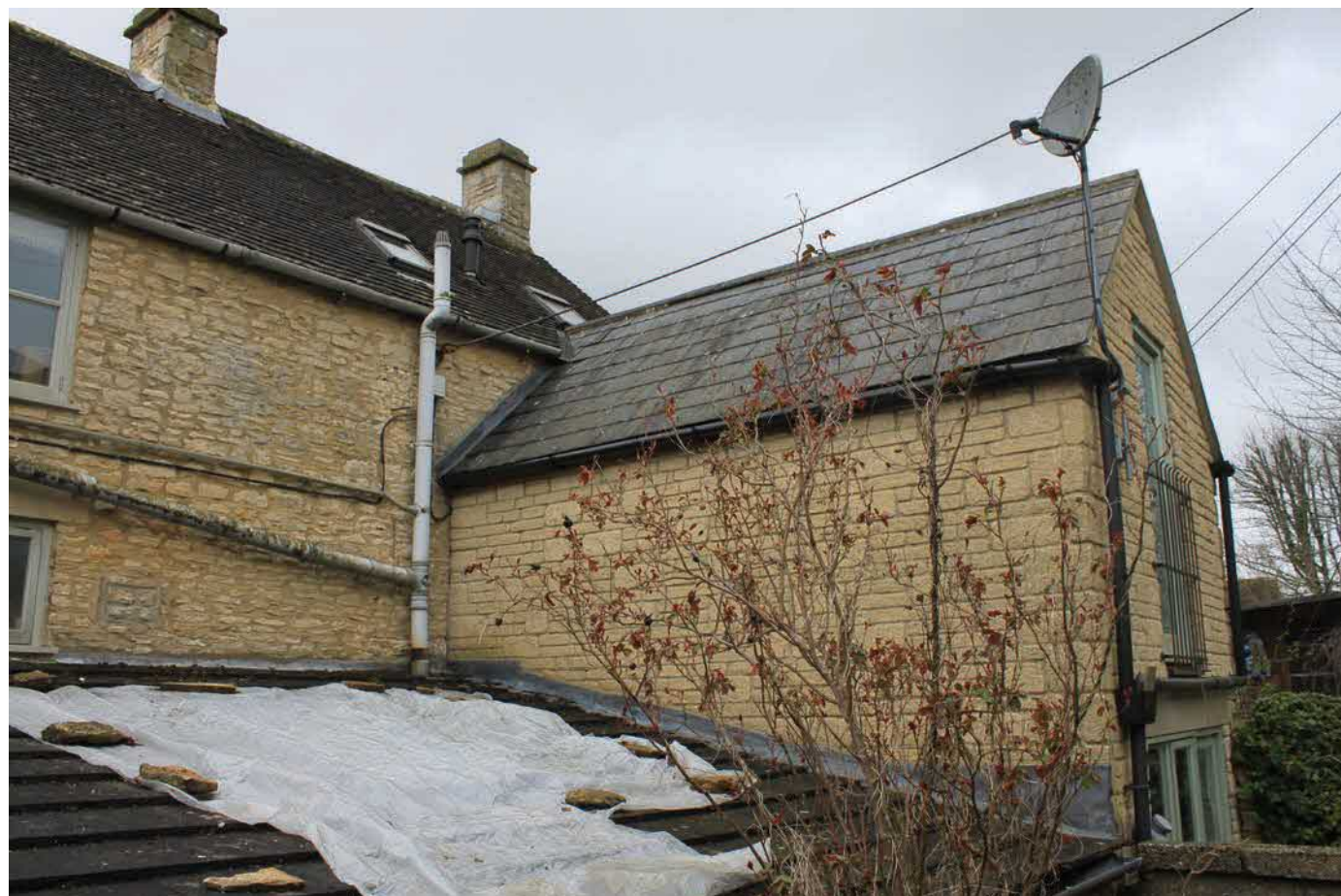
Single storey kitchen roof to rear and neighbouring two storey extension.
