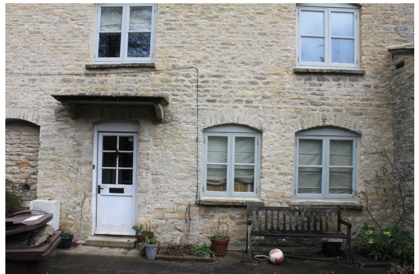
Front elevation showing the ground floor.
