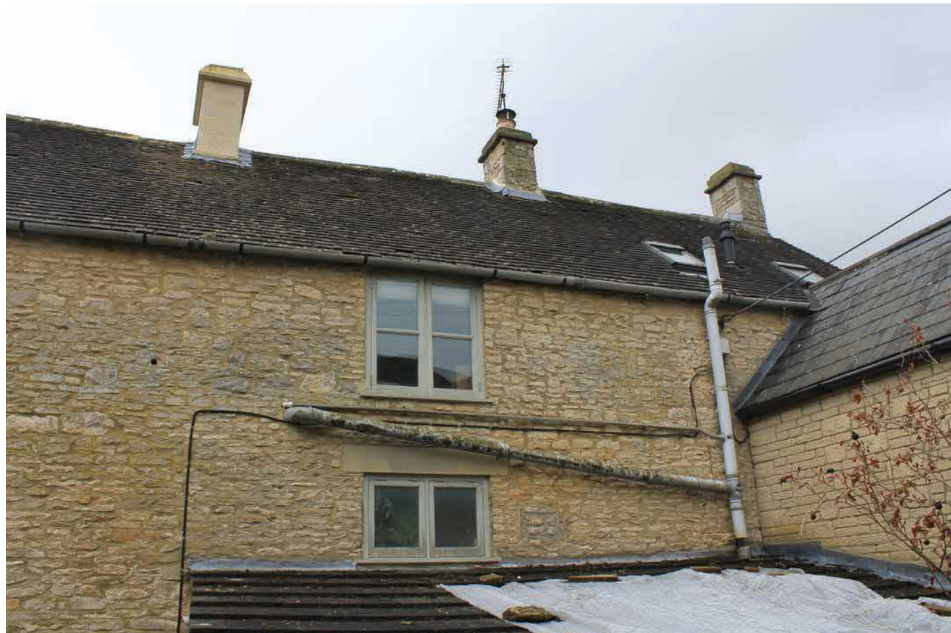
Rear elevation of upper floors.
