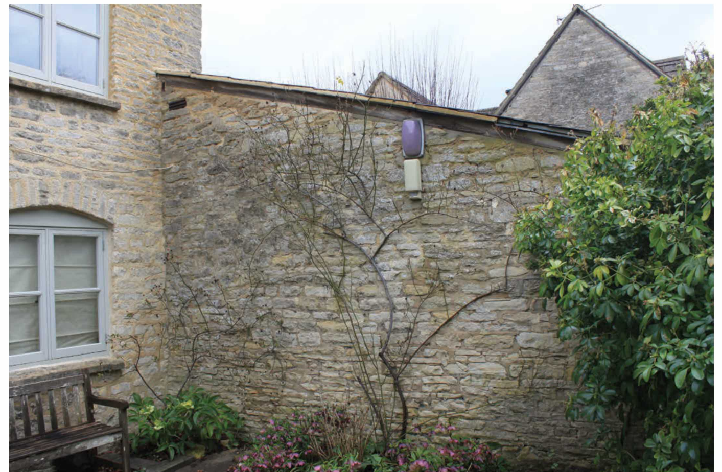
Side elevation of existing garage from the front courtyard.
