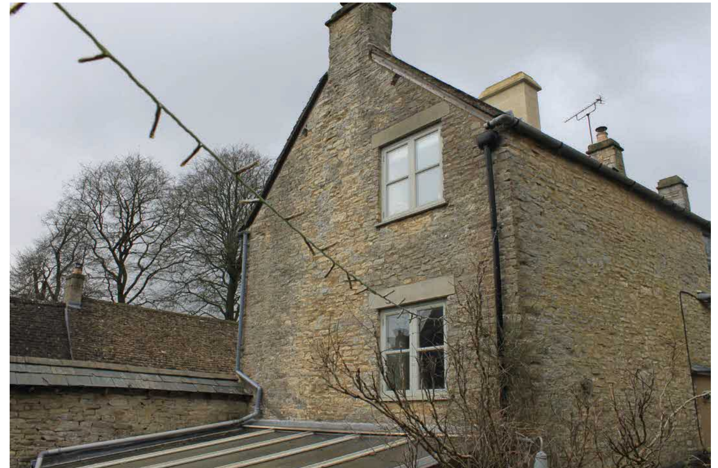
Side elevation of property from the garden.
