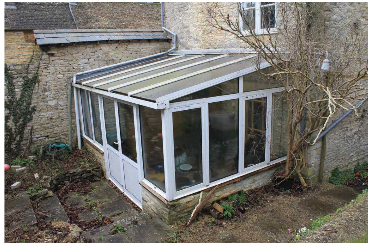
Existing side conservatory proposed to be demolished.
