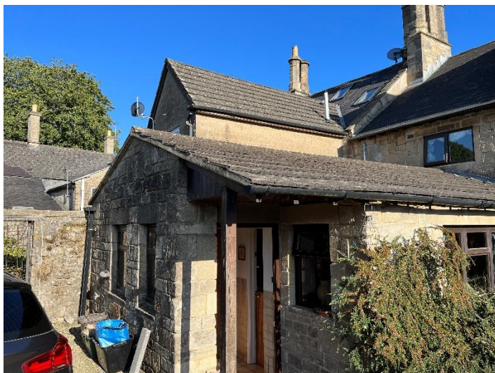
Figure 5: External view of kitchen and utility building of the main house
