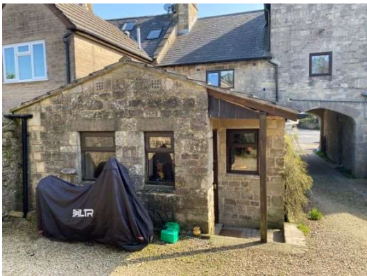
Close up looking North of existing kitchen Extension.
