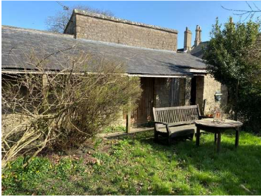
North corner of outbuilding to left, existing kitchen extension to right
