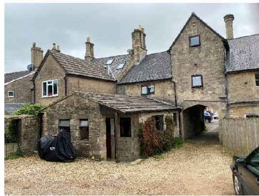
View South back towards existing house.
