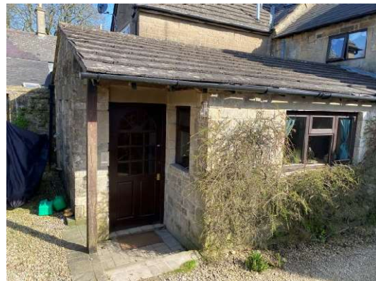
West elevation of existing kitchen extension.
