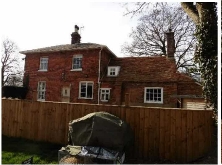
Millers east façade
