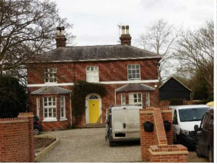
millers north façade
