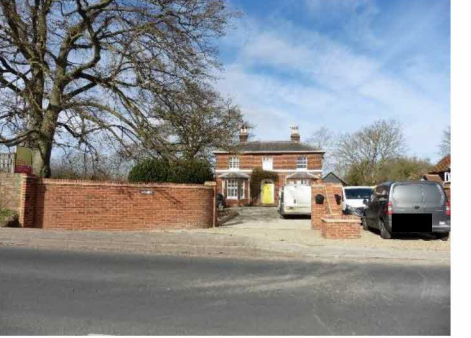
millers north façade
