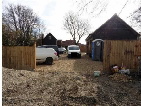
Stables north façade and outbuilding
