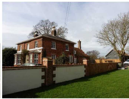
Millers south and east façades
