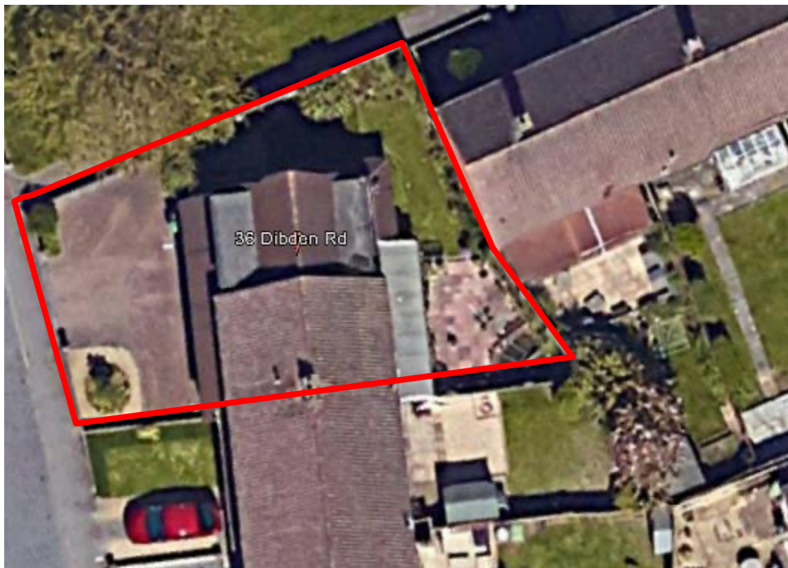
Fig.3. Google earth Aerial View of Dibden Road with the site highlighted
