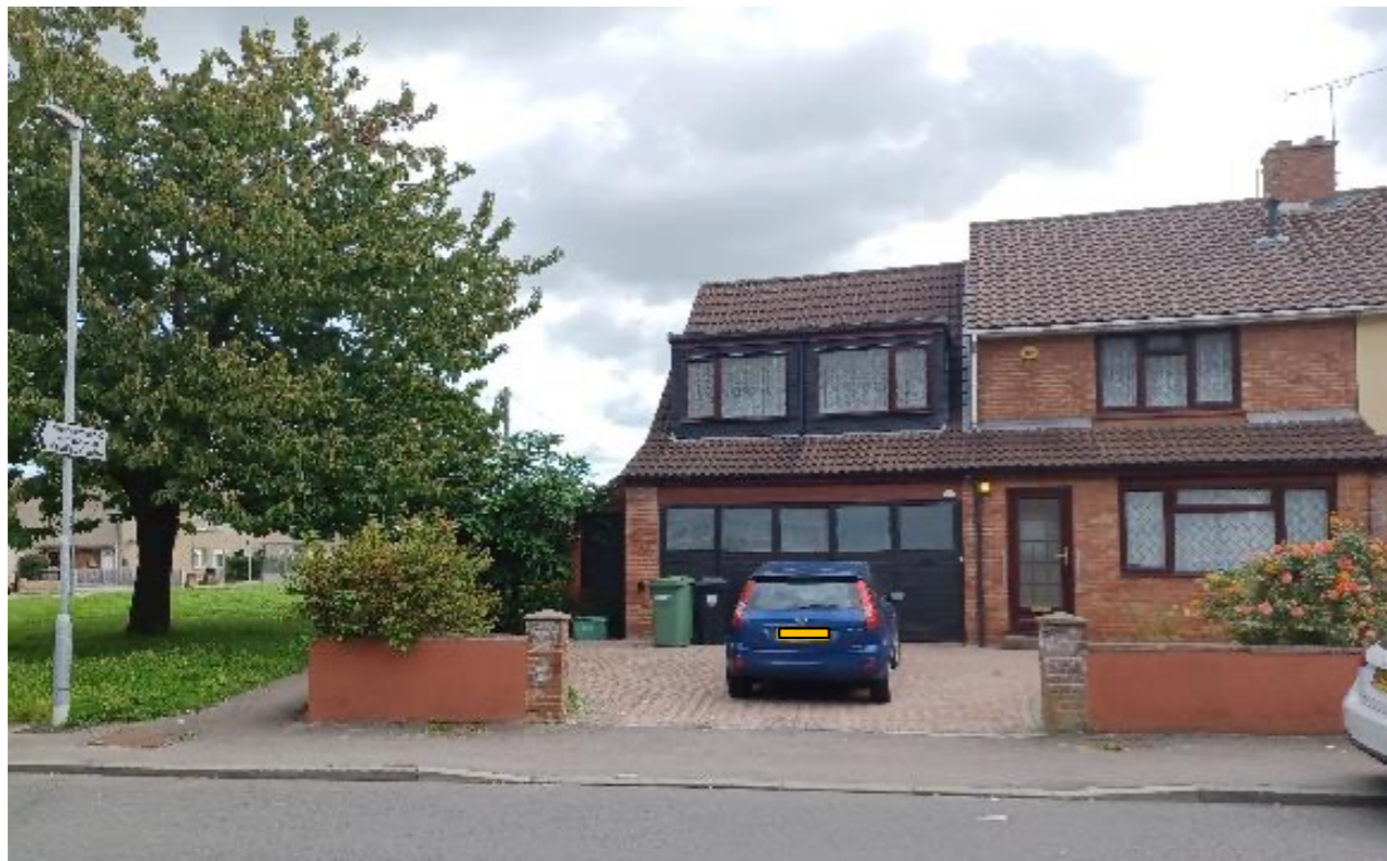
Fig.5. Entrance to application site from Dibden Road
