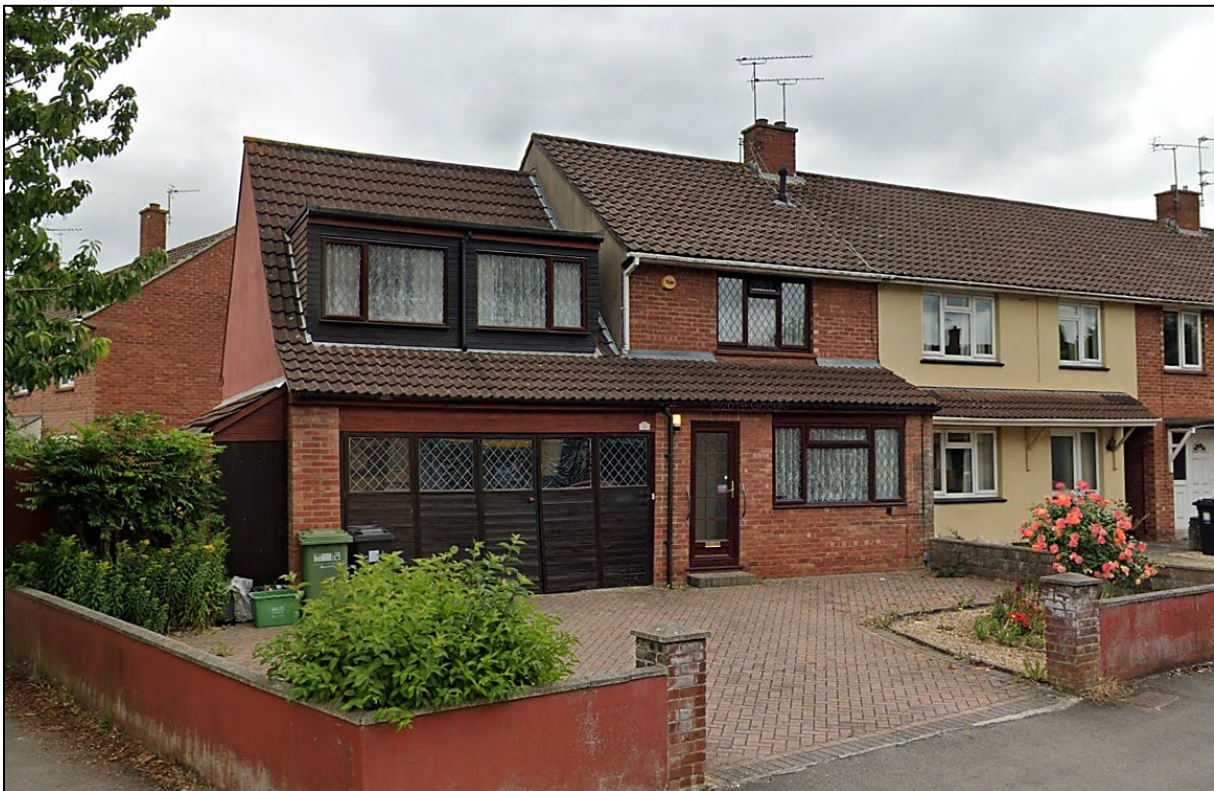
Above - Application site viewed from Dibden Road
