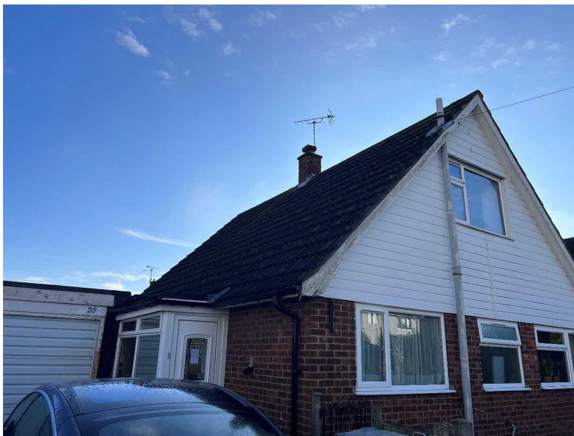
Photograph 2: The west and north elevations of the building.
