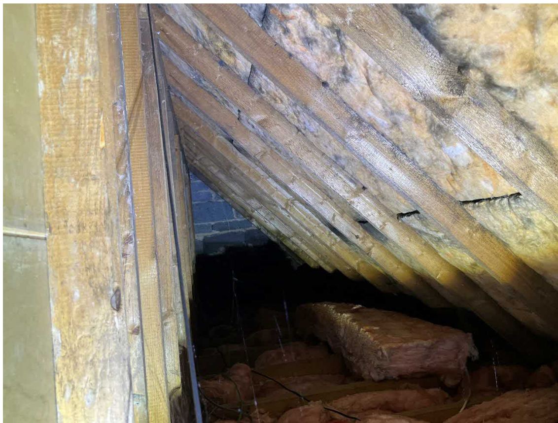
Photograph 4: The internal roof structure.
