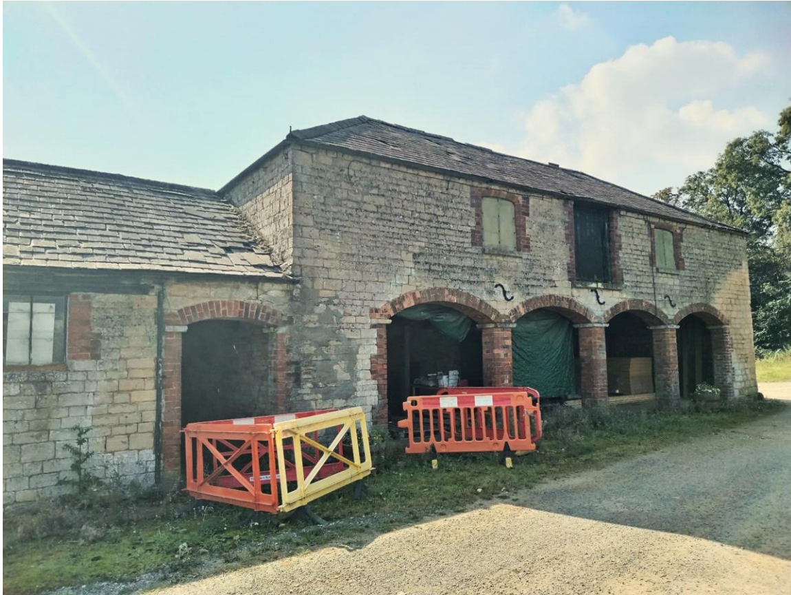
(Above) The existing front of the building (North Facing)
