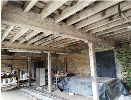
(Above) All existing timber beams, posts and king post trusses to be retained and left exposed.
