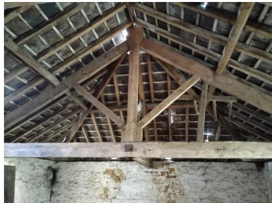
(Above) All existing timber beams, posts and king post trusses to be retained and left exposed.
