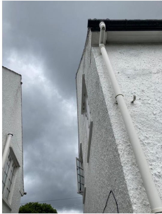
Corbell at eaves
