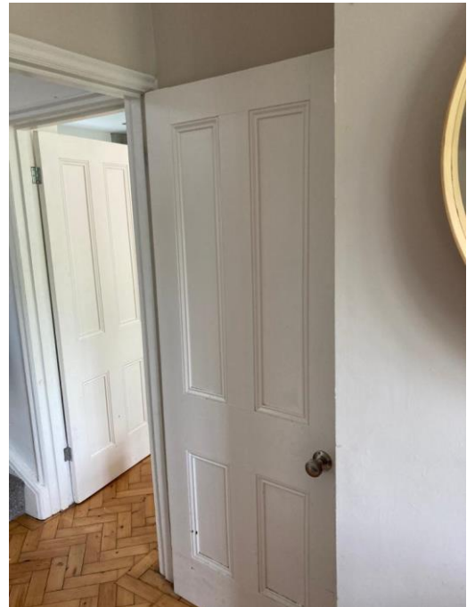
Four-panelled doors throughout
