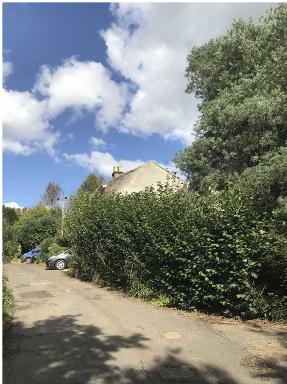
South elevation from Frank's Hollow Road
