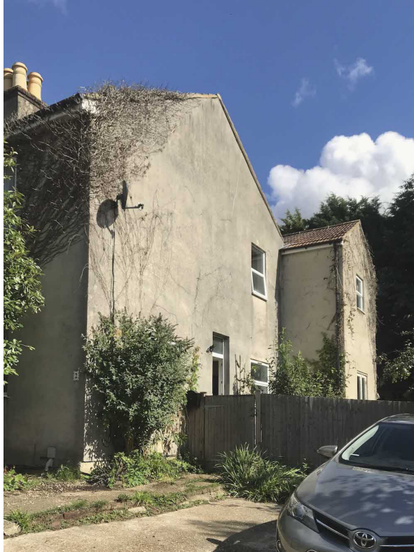
South-west elevation showing extent of two-storey extension from Frank's Hollow Road
