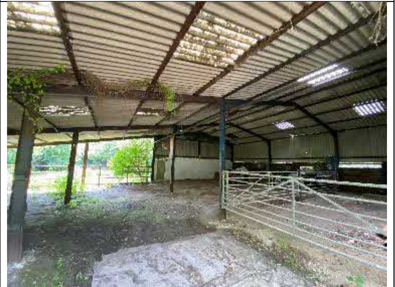
Figure 8 Interior of B1.
