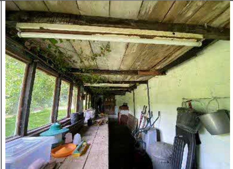
Figure 9 Interior of the single storey extension of B1.
