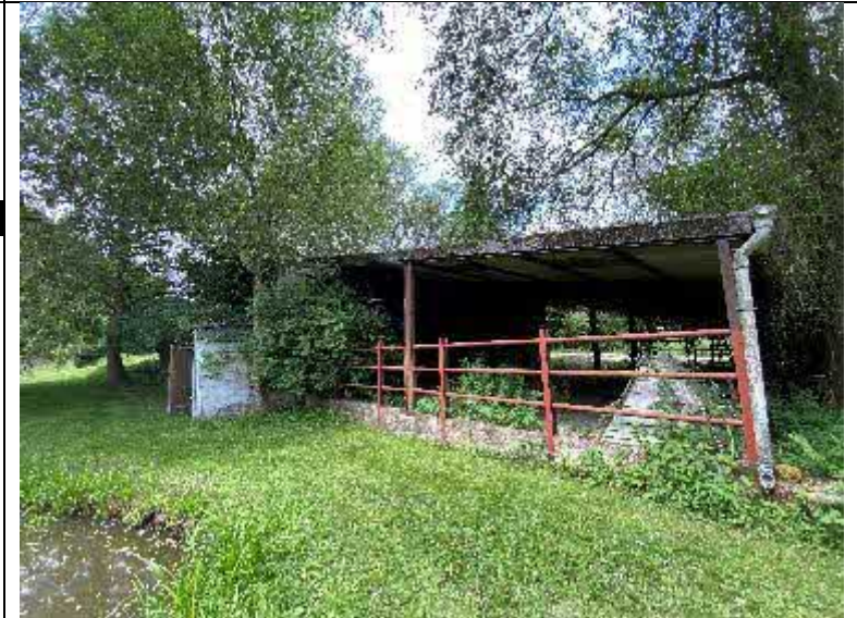
Figure 5 South-eastern elevation of B1.
