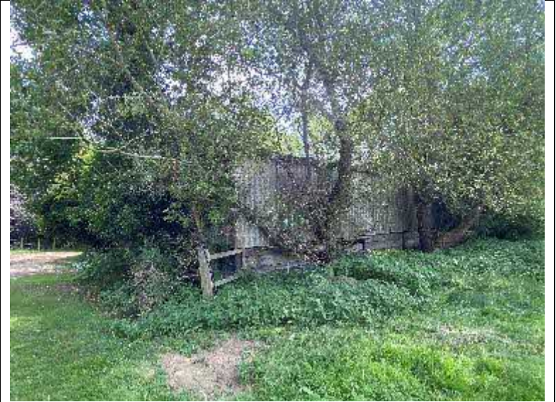
Figure 7 South-western elevation of B1.
