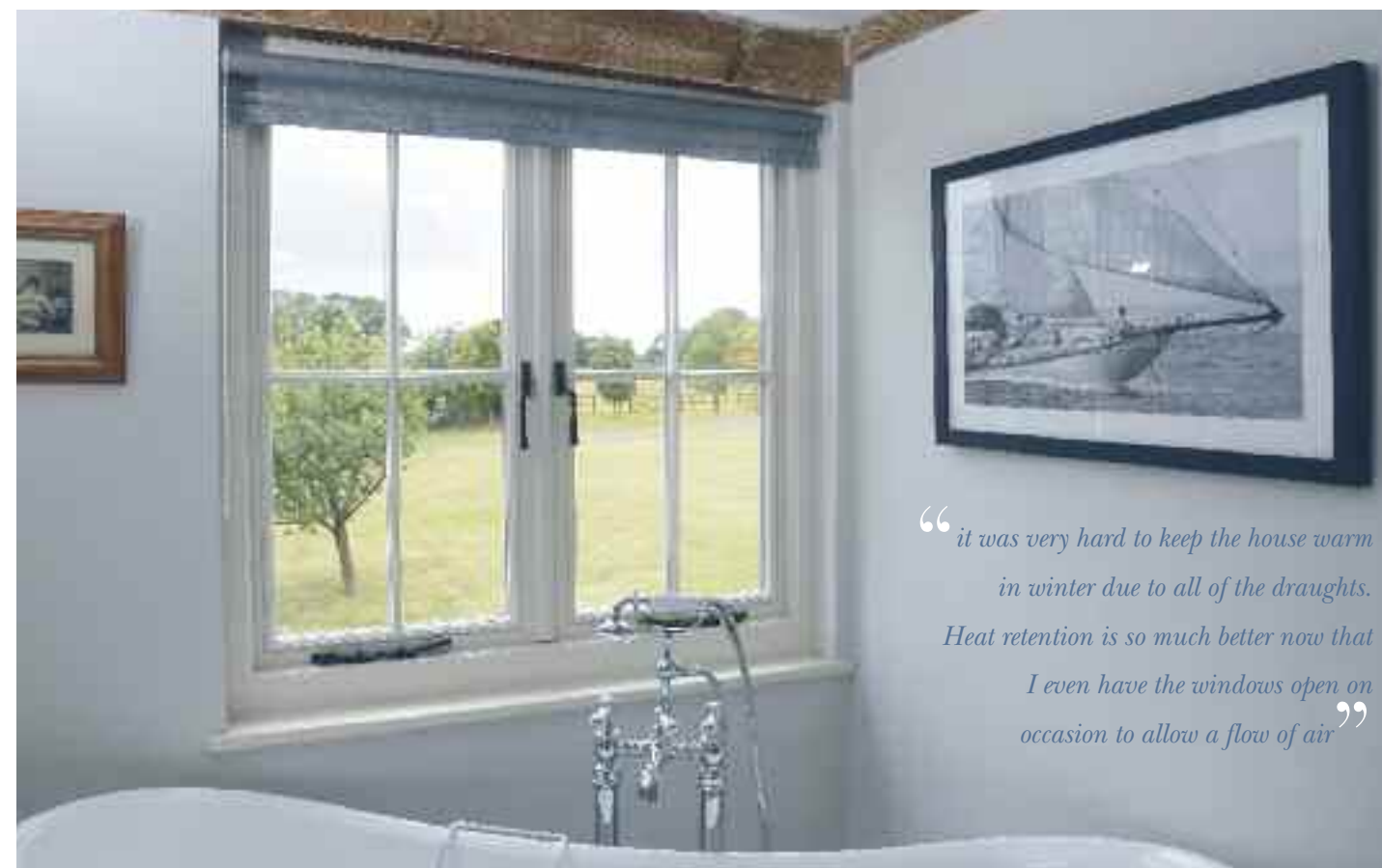
Cream cottage flush casement with 18mm astragal bars.
