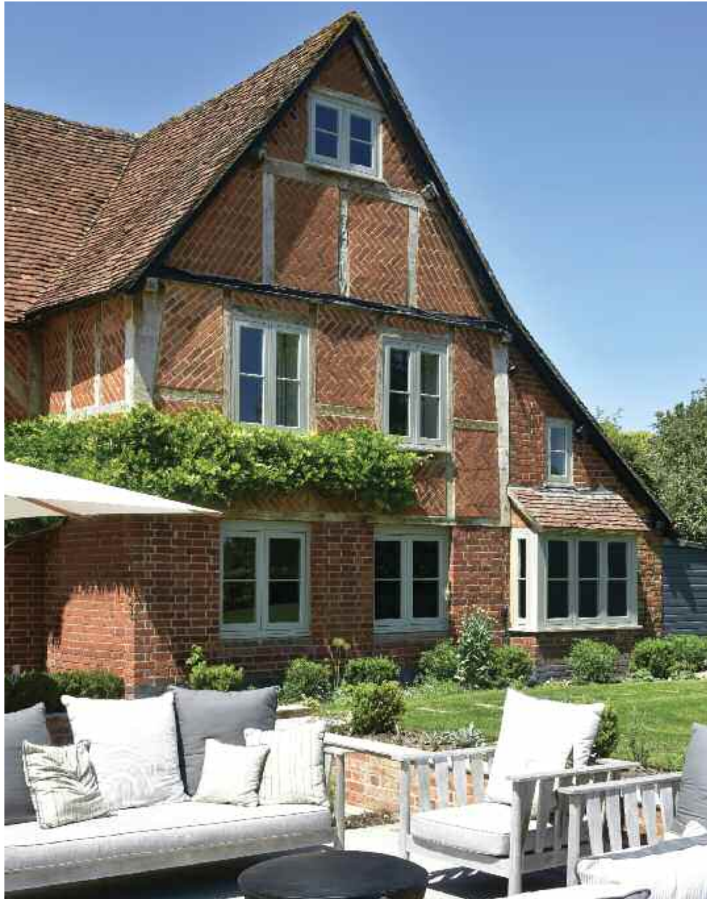
Listed flush casements with 22mm true bars in a colour complementary to Farrow & Ball 'Hardwick White'.
