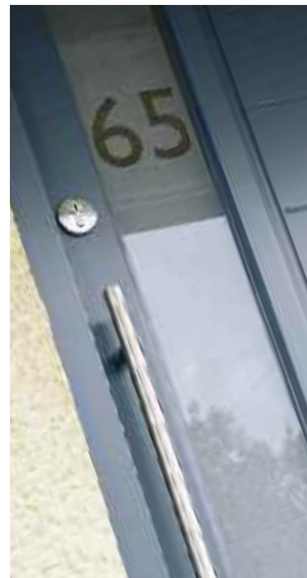
TOP Peater Shakespeare knocker and Bright Star glass. MIDDLE Sandblasted glass with etched house number and Polished Chrome Samuel Heath Ring knocker. LOWER LEFT Antique Brass Unlacquered Medium sized Samuel Heath letter plate. LOWER MIDDLE Polished Chrome Reeded handle. LOWER RIGHT Sandblasted glass with etched house number, with 316 Coastal Grade Stainless Steel contemporary Guardsman handle.
