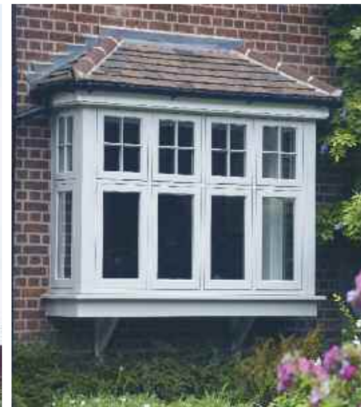
Porcelain flush casements with 18mm astragal bars.
