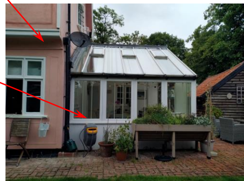
Figure 7 – View of existing Conservatory
