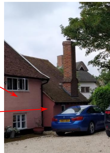
Figure 5 – View of existing Garden Room from North East
