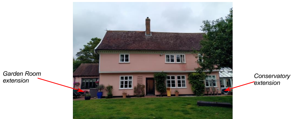
Figure 3 – View of existing dwelling from South
