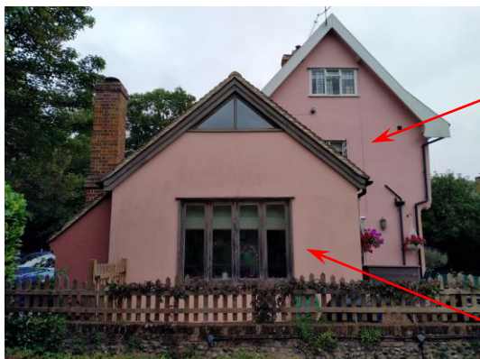
Figure 4 – View of existing Garden Room from West
