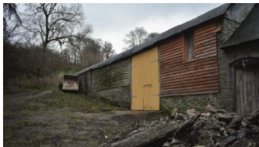
Fig.31. North elevation of barns 5 and 6
