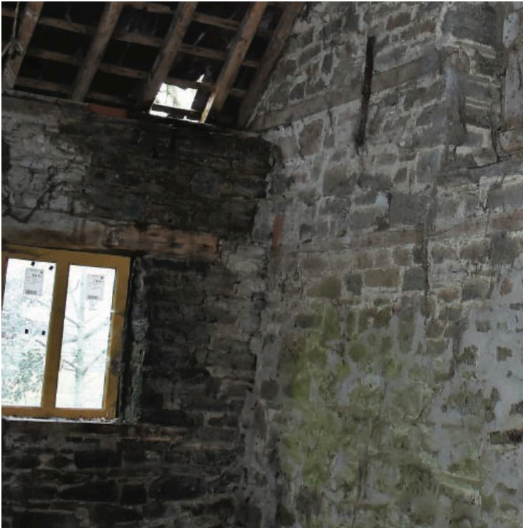
Fig.29. Interior of north west corner of barn 4 showing the north wall as a later build.
