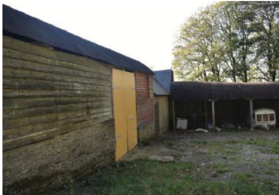
Fig.37. Eastern elevation of barn 7
