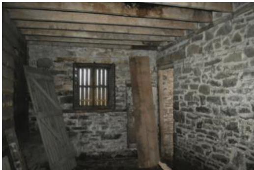
Fig.24. Interior of one of the loose boxes with concrete corner feature
