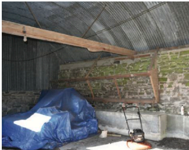
Fig.35. North elevation of barn 6
