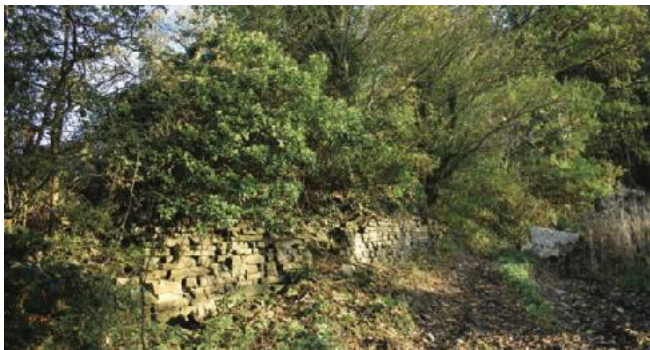
Fig.6. The remains of the demolished stone barn to the south of Old Burfa
