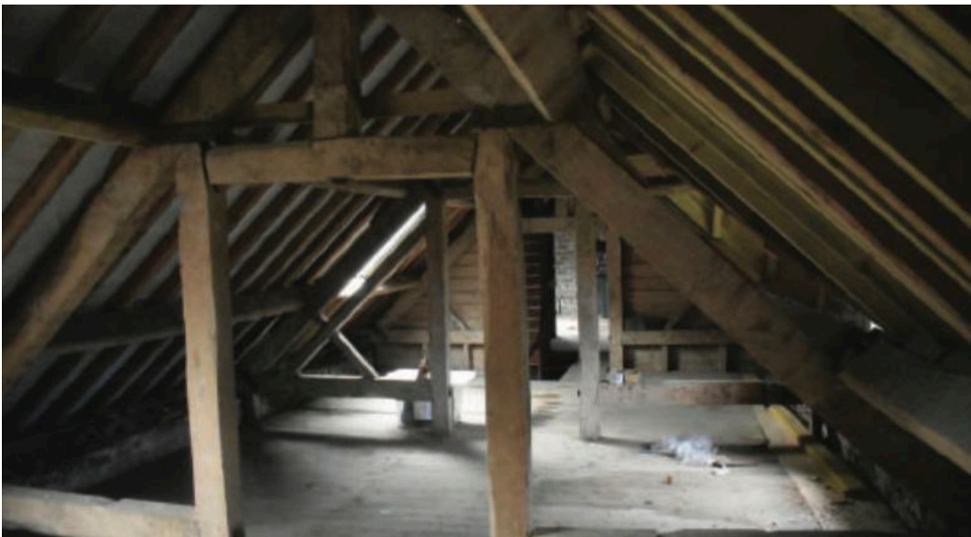
Fig.20. View of upper floor barn 2
