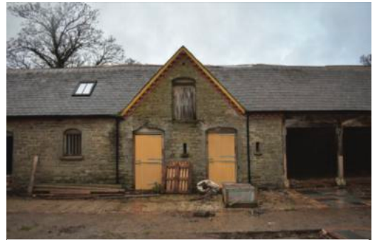
Fig.23. East elevation of barn 3
