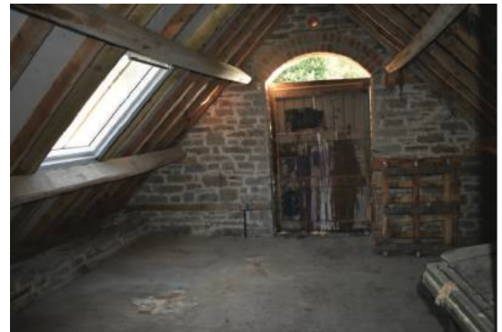
Fig.14. The upper floor of Barn 1, previously the granary
