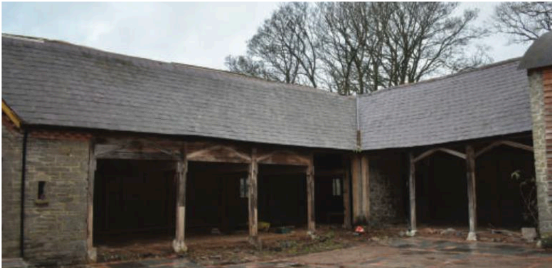
Fig.30. Courtyard elevation of barn 4
