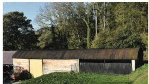
Fig.32. South elevation of barns 5 and 6
