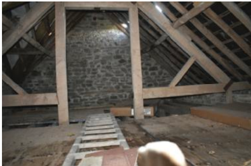
Fig.22. Upper floor of barn 3, looking south from doorway to barn 4
