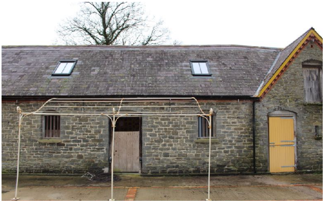
Fig.4. Yard side elevation showing timber louvred windows of barn 2
