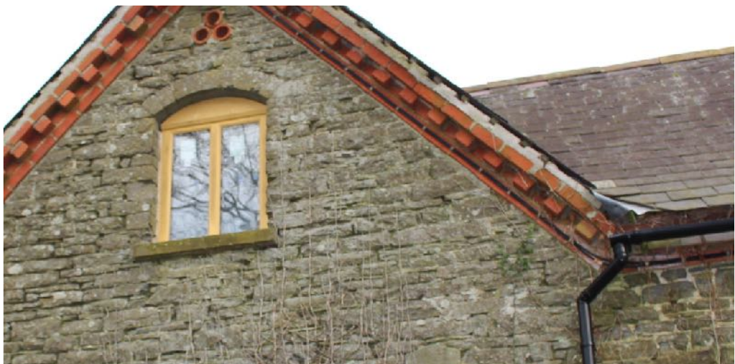
Fig.2. Window installed without LBC on western elevation of barn 3
