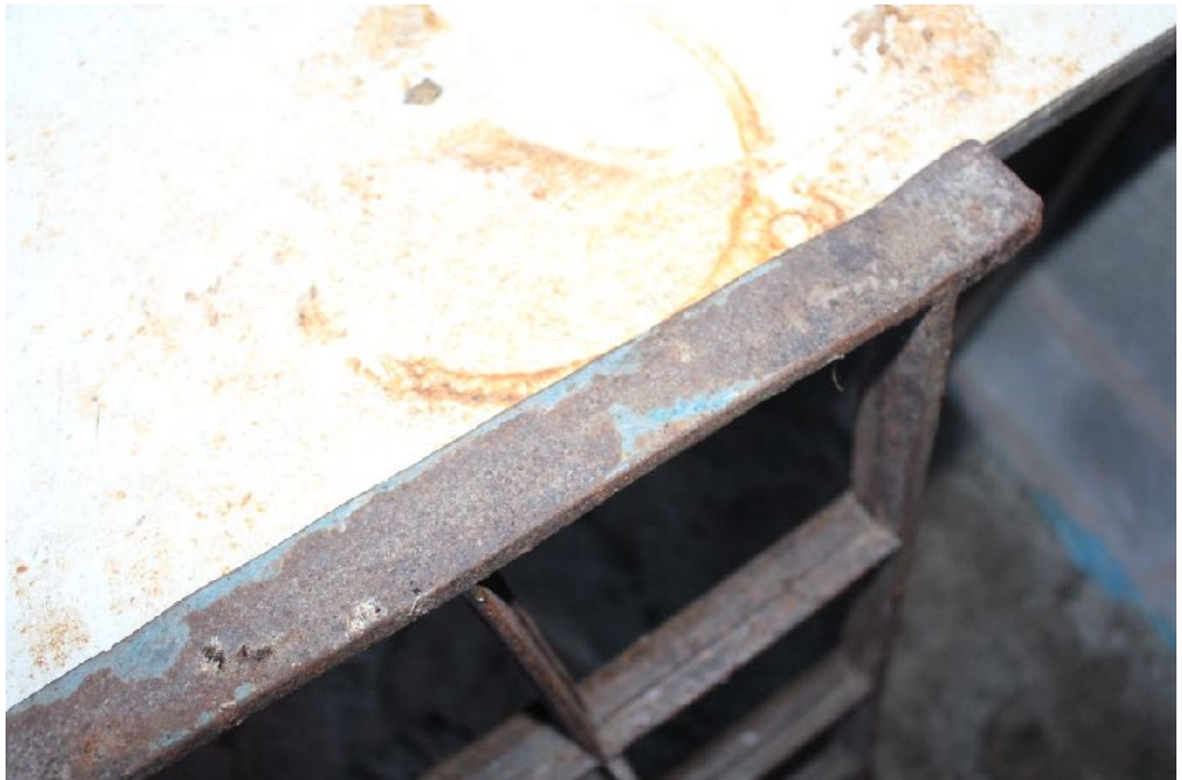
Fig.10 Close up of surveying paint flecks on metal frames.
