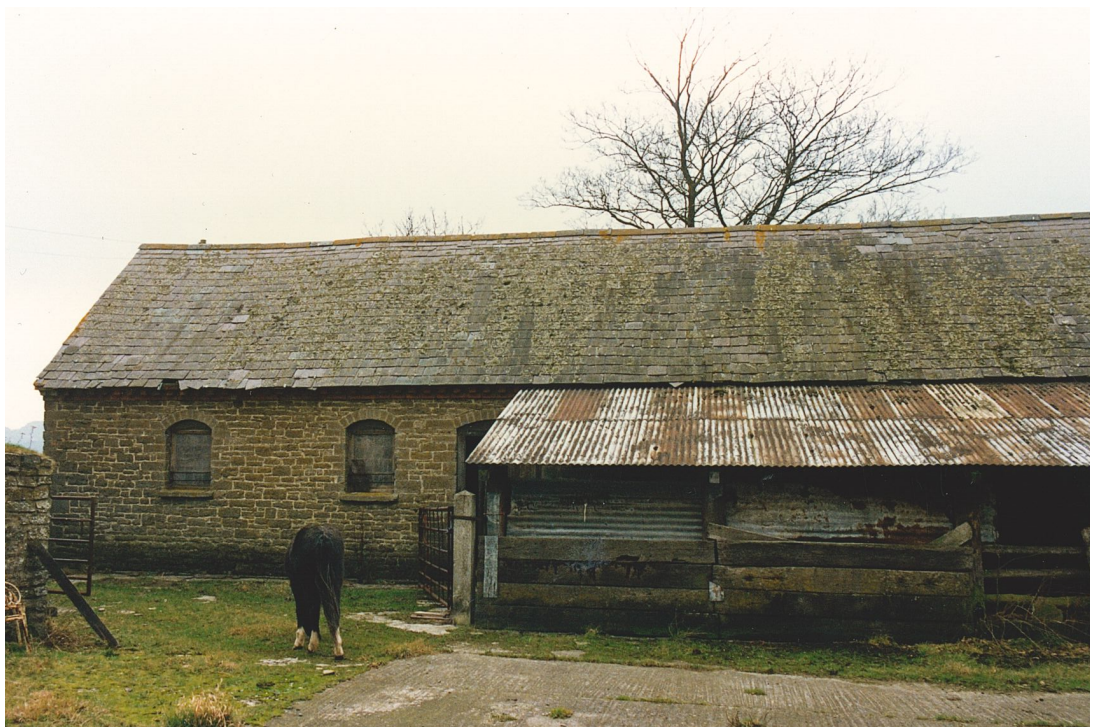
Fig.3. Cadw photo from 1992 Listing showing metal frame windows and now demolished outshut.
