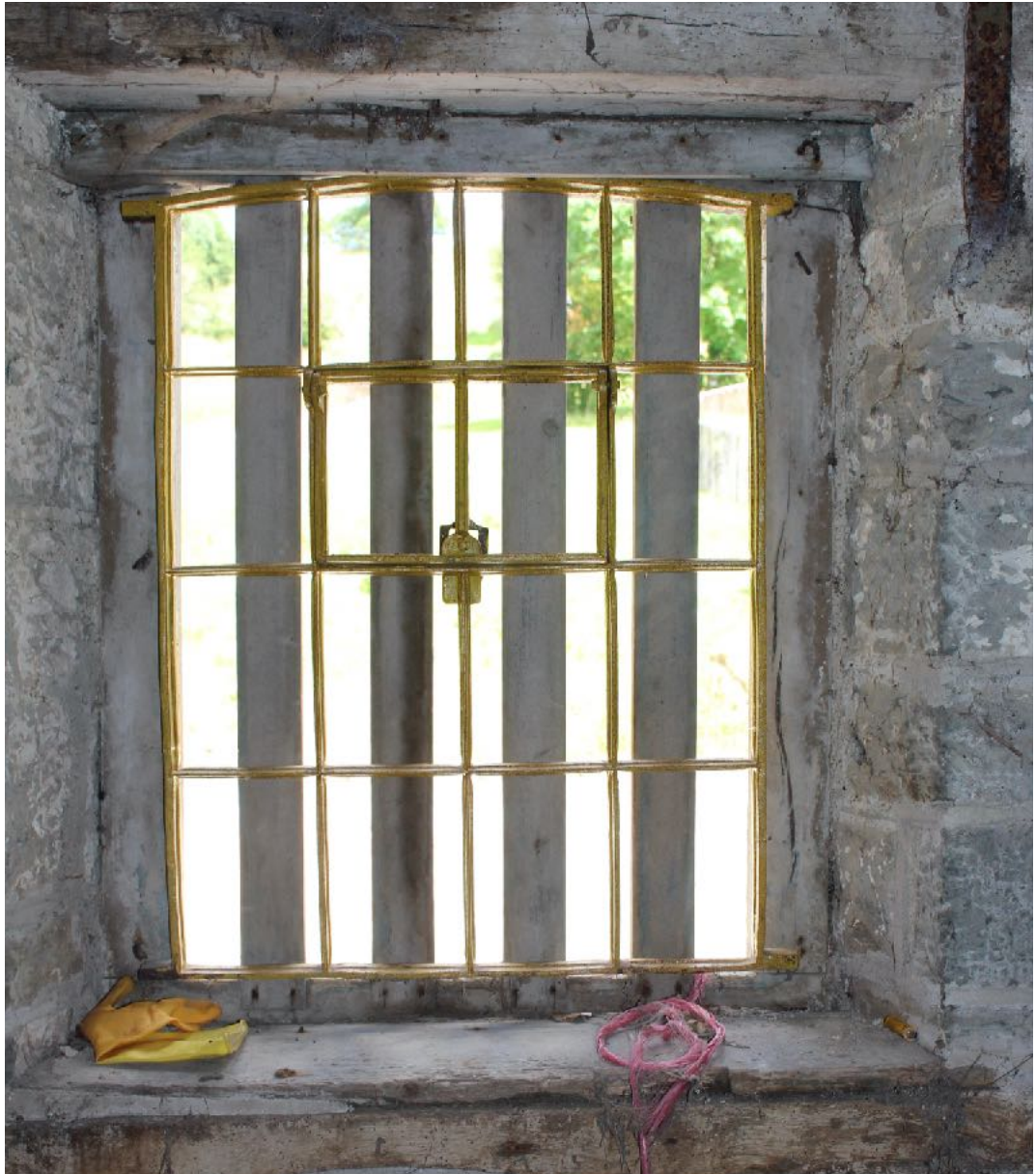
Fig.7. Barn 2 timber louvred window from inside with metal frame placed over.
