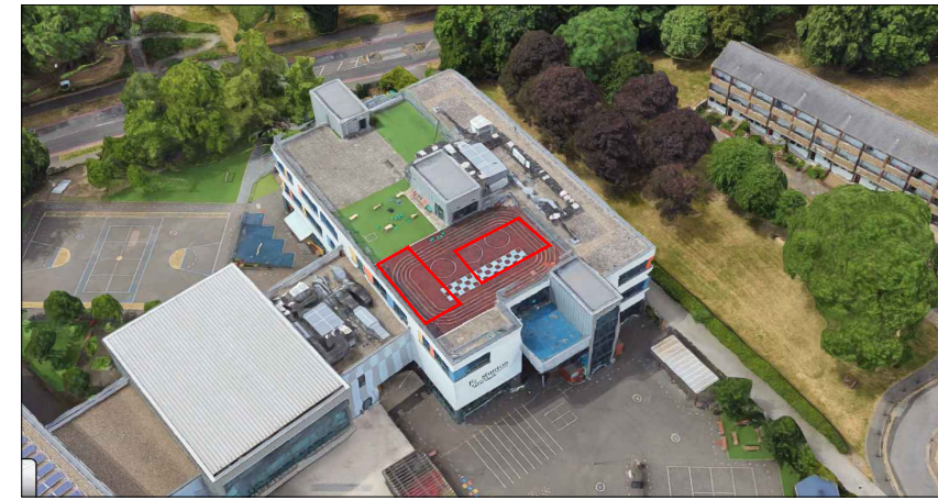
ASHP Enclosure Location
