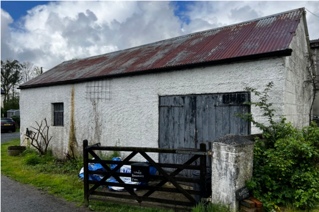
Plate 2. Eastern elevation of barn
