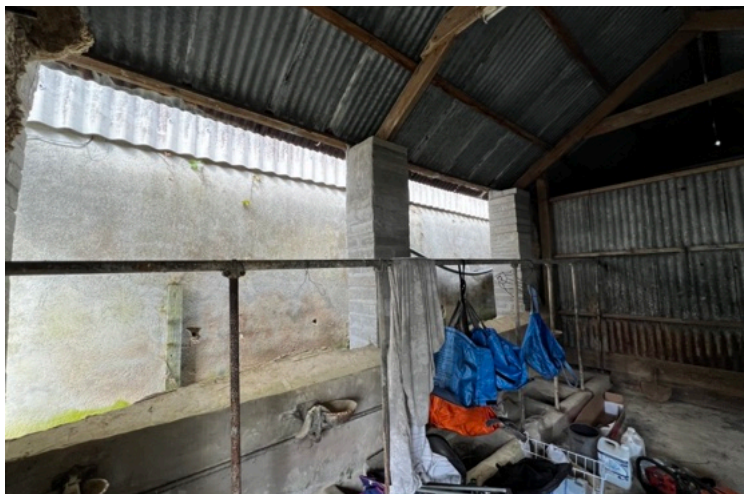
Plate 5. Internal view open to most of the western elevation
