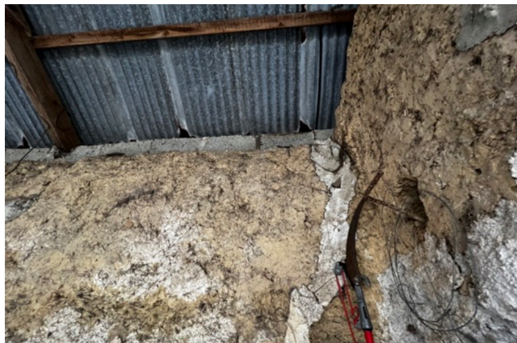
Plate 6. Corrugated sheet roof and cob wall sections
