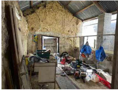
south area of barn
