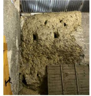
The remaining sections of cob walling are in extremely poor condition, especially at the base, where there is evidence of erosion possibly caused by livestock rubbing up against the walling. There is also severe burrowing by vermin. This may explain why some sections of the cob walling have been lined with concrete blockwork at the base. Photograph opposite shows failing cob at base of wall.
