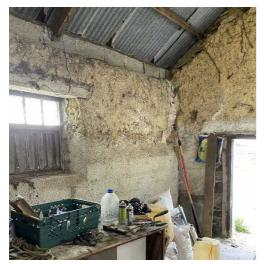
The photograph (left) shows the concrete block lining to the base of the remaining cob walling. 2.06b Condition cont....
