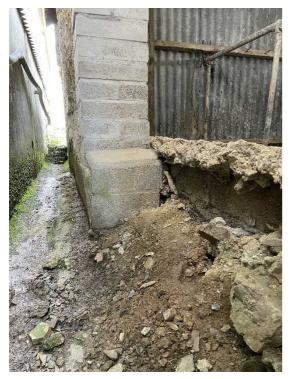
The concrete blockwork to the piers on the West elevation appears reasonably 'fresh'. Either side of the central pier there are the remains of cob walling at low level. This suggests, this wall was once cob and continuous to form an enclosed structure building, with the piers being constructed post collapse. Photograph opposite (left) shows remains of collapsed walling.
