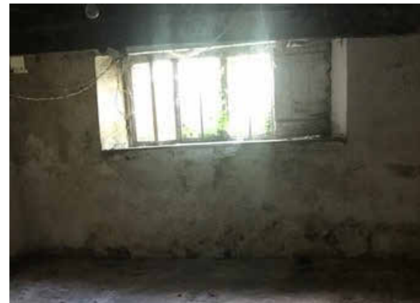
Annex internal view
