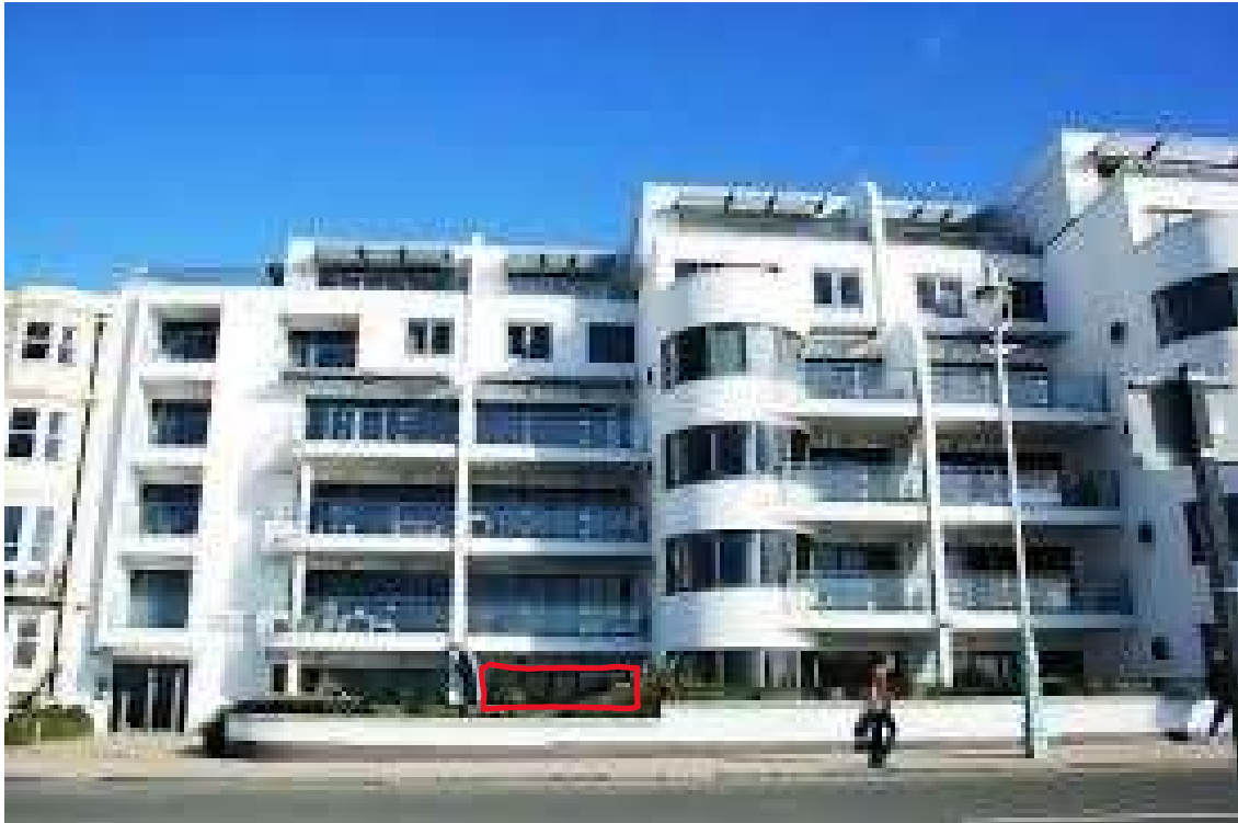
Front elevation of the Van Alen Building, BN2 1WP showing proposed position of 6 panel replacement windows for Flat 23, in red.
