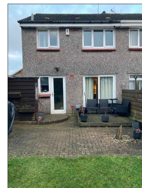
PHOTO EXISTING WEST ELEVATION
