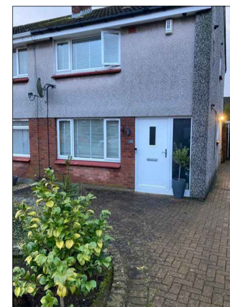
PHOTO EXISTING EAST ELEVATION
