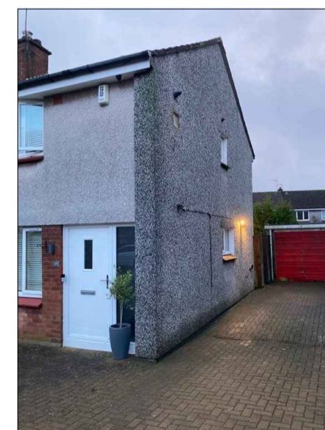
PHOTO EXISTING NORTH ELEVATION
