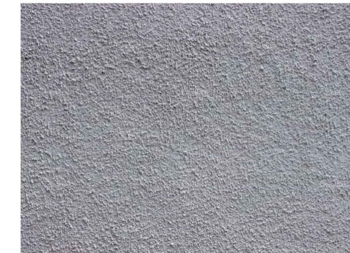
White wet-dash Render to match the existing house and extension.
