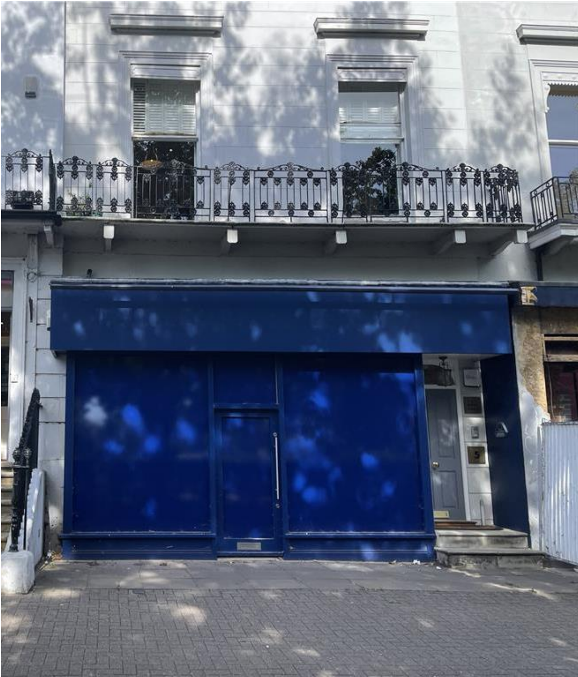
(1) Photograph of shop front prior to change
