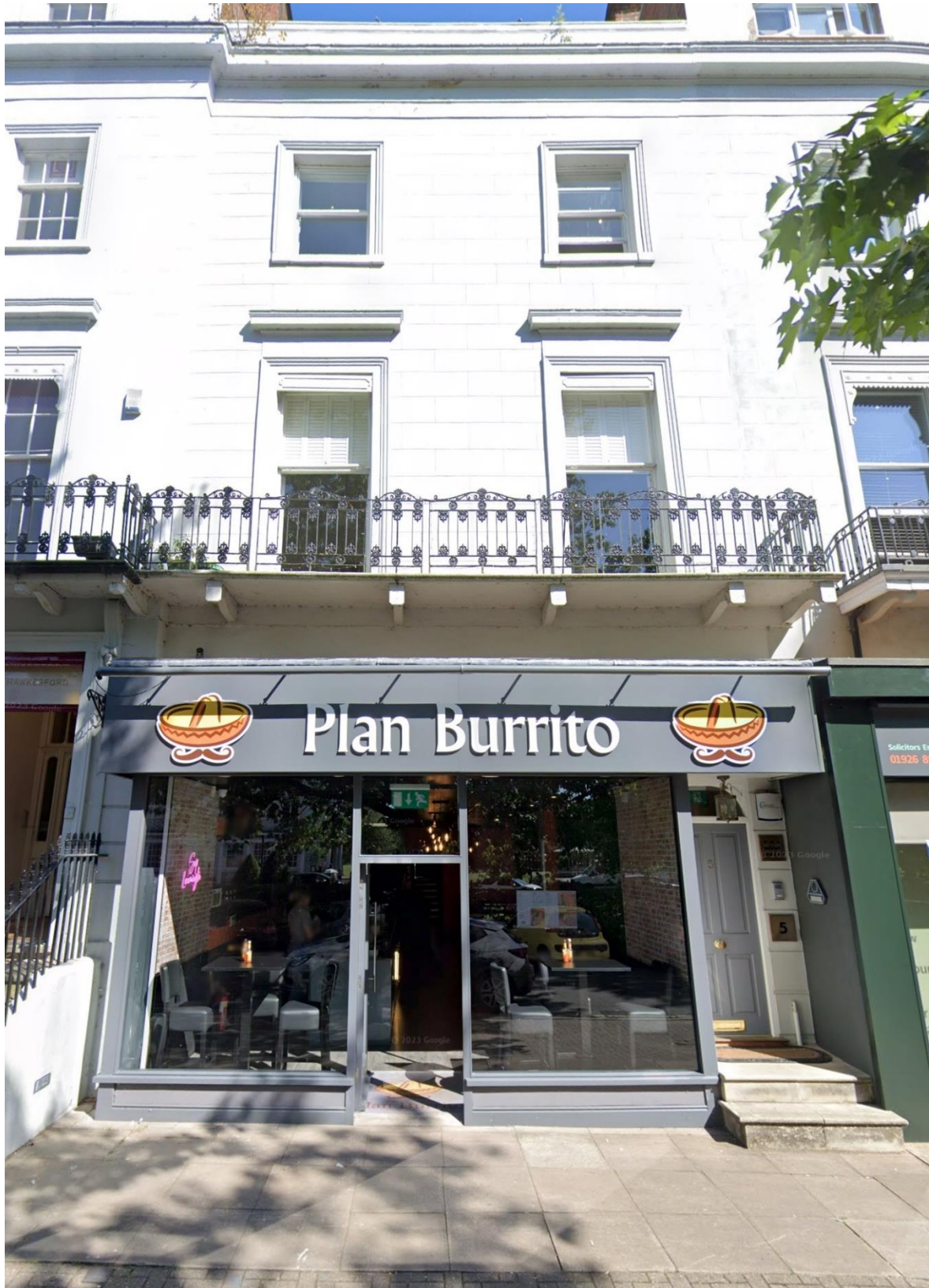
(2) Photograph of shop front current, after change
