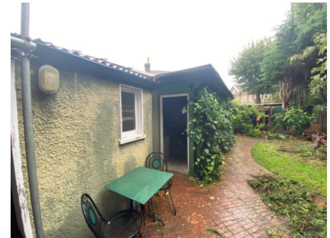
The rear extension and garage
