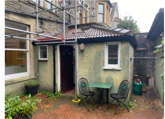
20 Blenheim Road, existing rear extension
