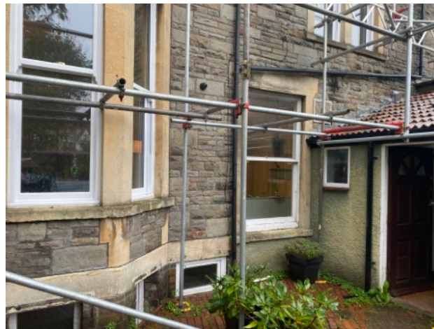
20 Blenheim Road, existing kitchen window
