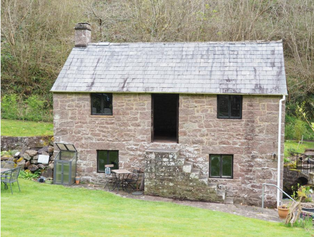
Plate 3: Cider Mill south elevation.
