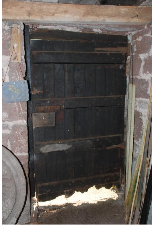
Plate 25: Cider Mill GF boarded and braced door from interior.
