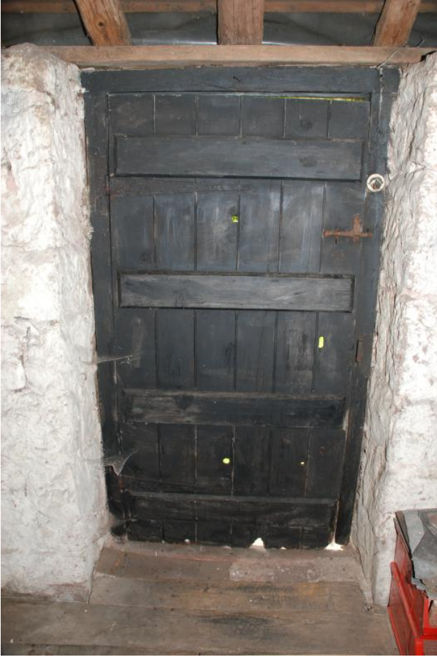
Plate 24: Cider Mill FF loft boarded and braced door from interior.
