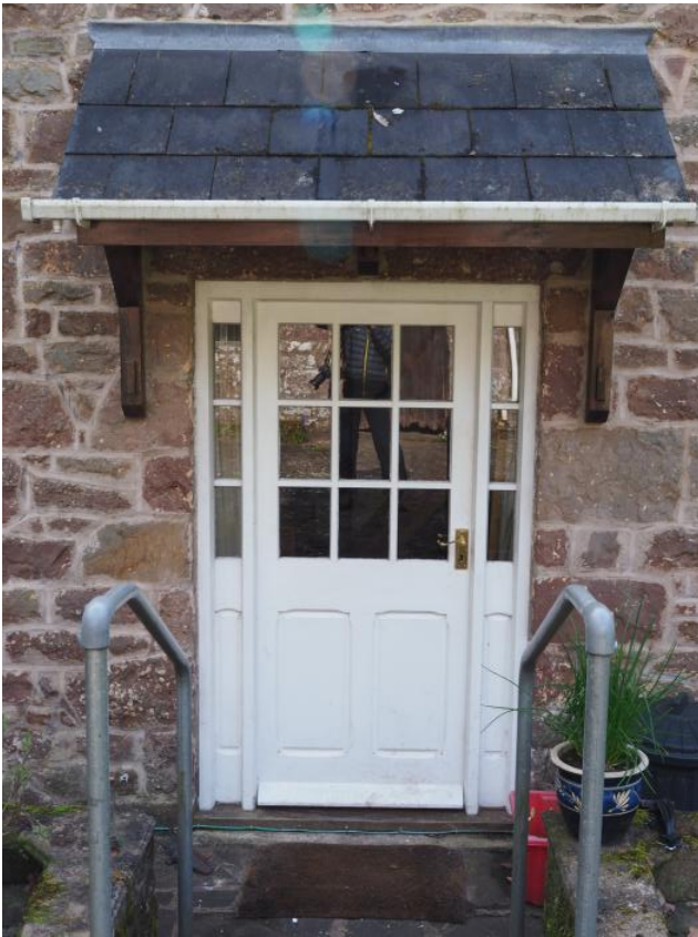
Plate 49: Cottage NW elevation door detail.
