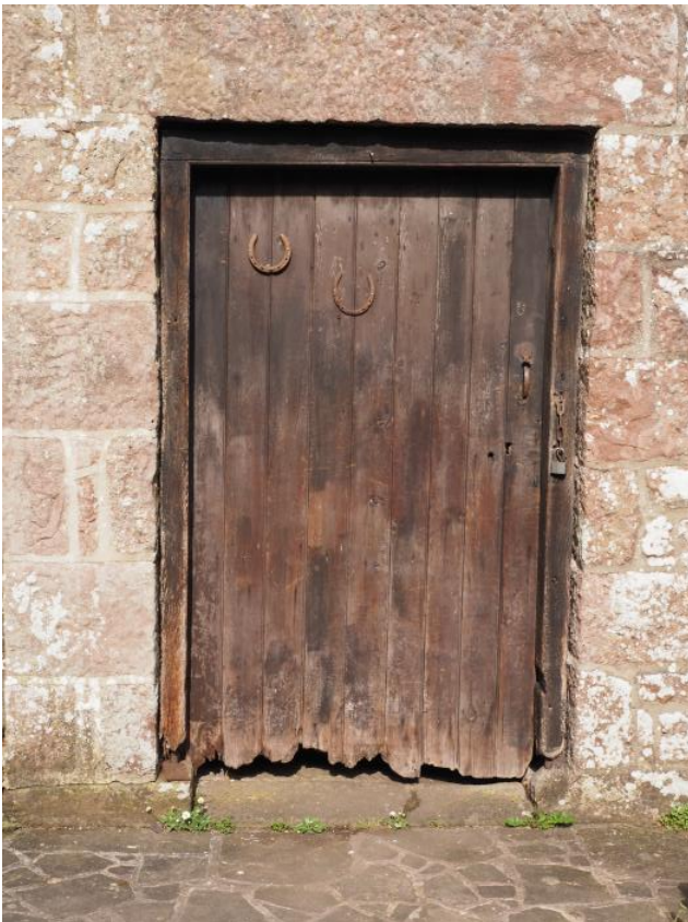
Plate 10: Cider Mill GF boarded and ledged door external.
