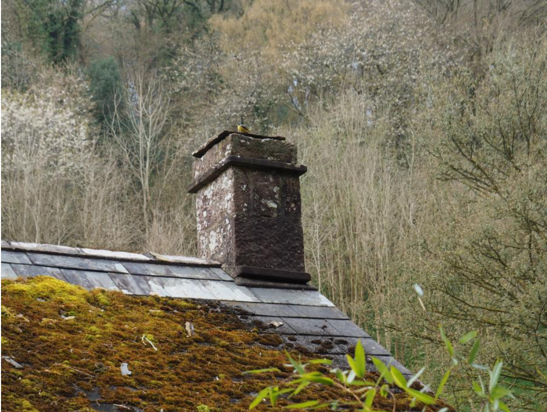
Plate 9: Cider Mill chimney stack/roof detail.
