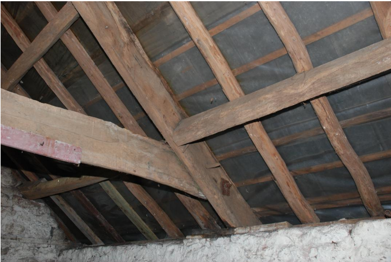
Plate 21: Cider Mill FF loft roof structure detail showing truss/purlin connections.
