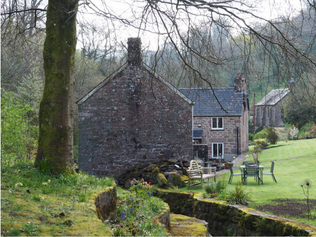
Plate 7: Cider Mill west elevation with cottage in background.
