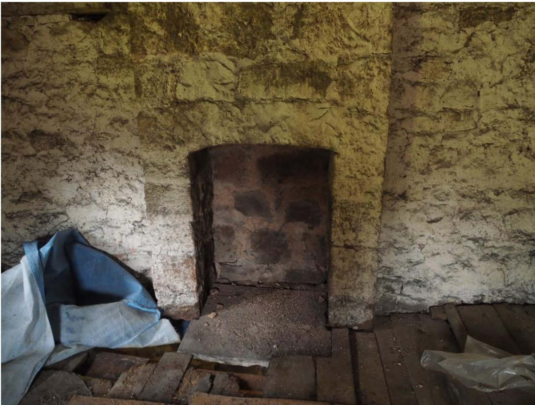
Plate 19: Cider Mill FF loft detail of fireplace and stone hearth.
