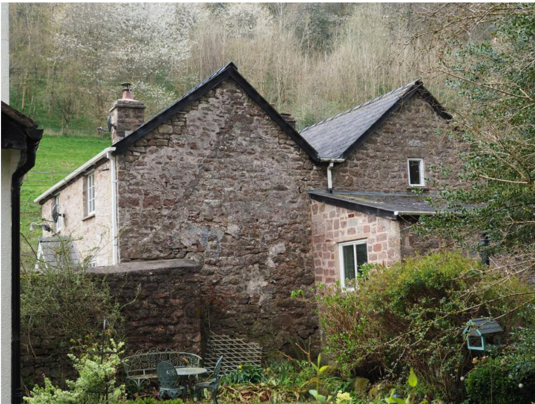
Plate 44: Cottage oblique view of north east elevation.
