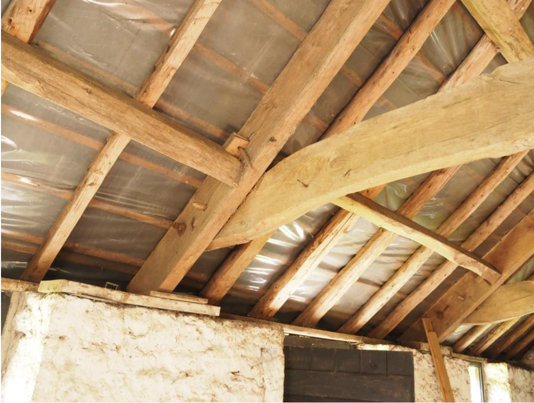
Plate 22: Cider Mill FF loft roof structure detail showing truss/purlin connections.
