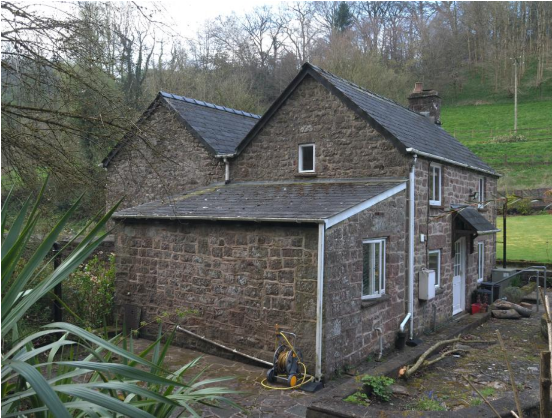
Plate 43: Cottage oblique view of north east elevation.
