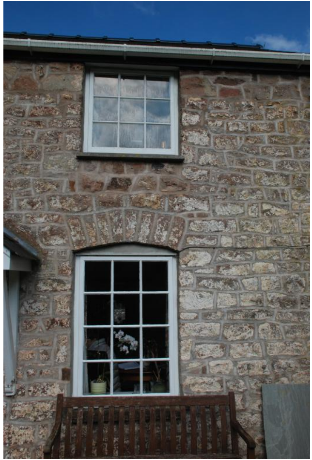
Plate 46: Cottage SW elevation timber windows.
