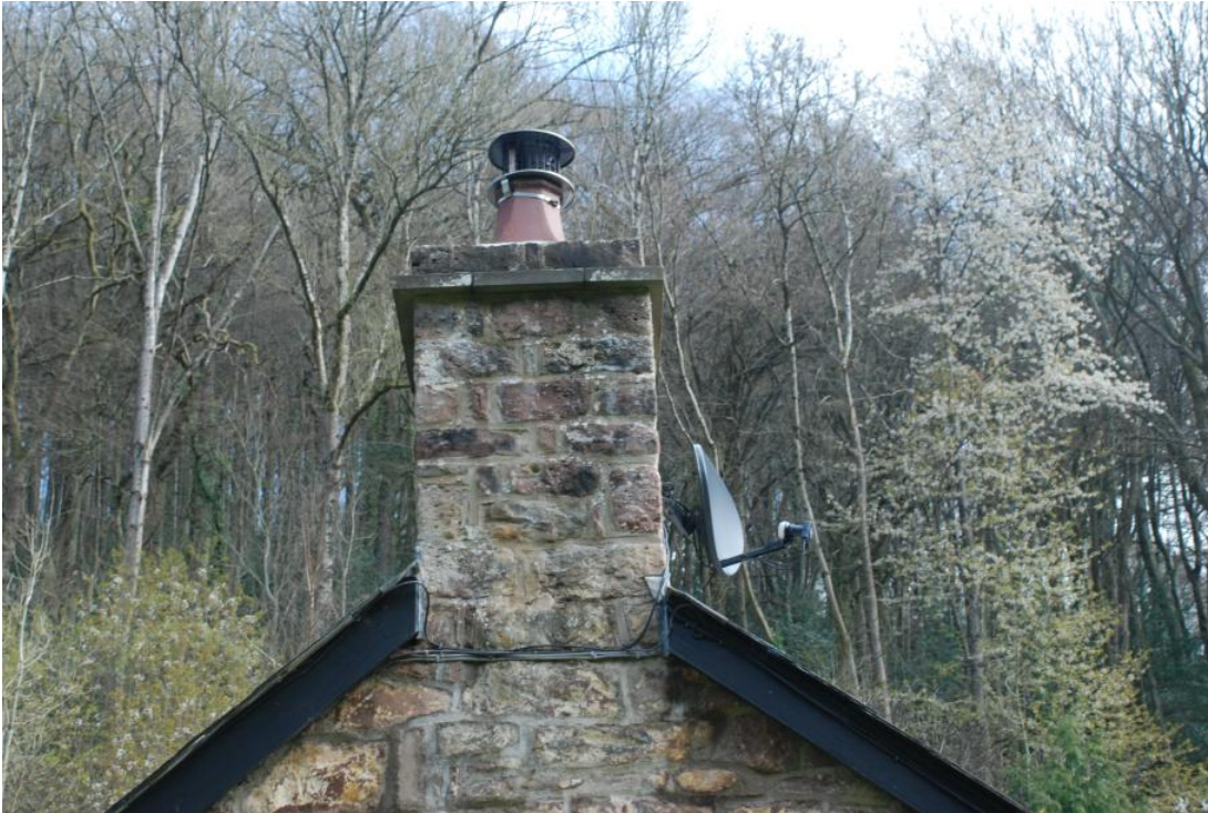
Plate 48: Cottage SW chimney stack detail.
