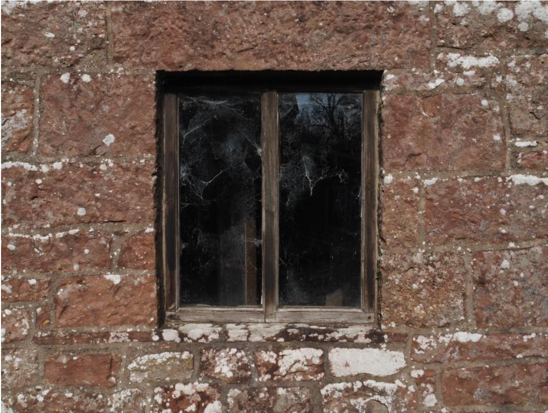
Plate 12: Cider Mill GF east gable window.
