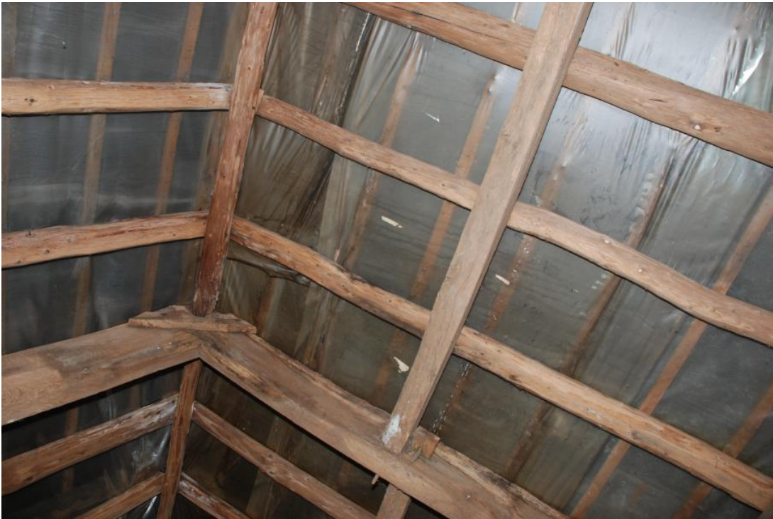
Plate 23: Cider Mill FF loft roof structure detail showing ridge.
