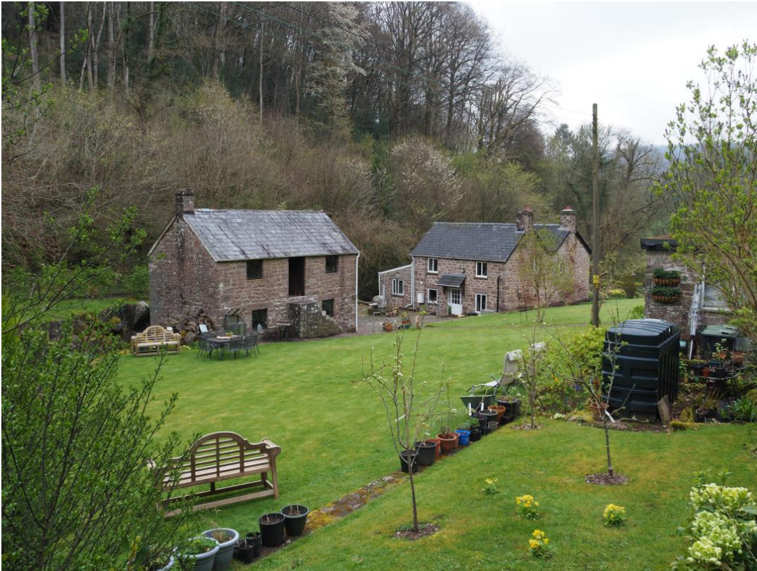
Plate 1: General view of building grouping from south west.
