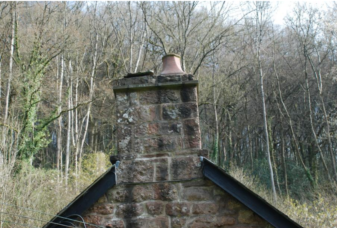
Plate 47: Cottage NW chimney stack detail.
