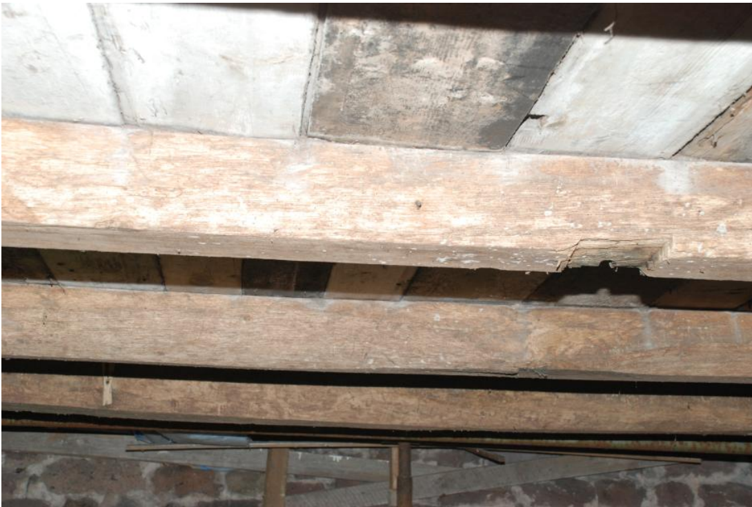
Plate 31: Cider Mill GF Cider House detail of FF beams and floorboards.
