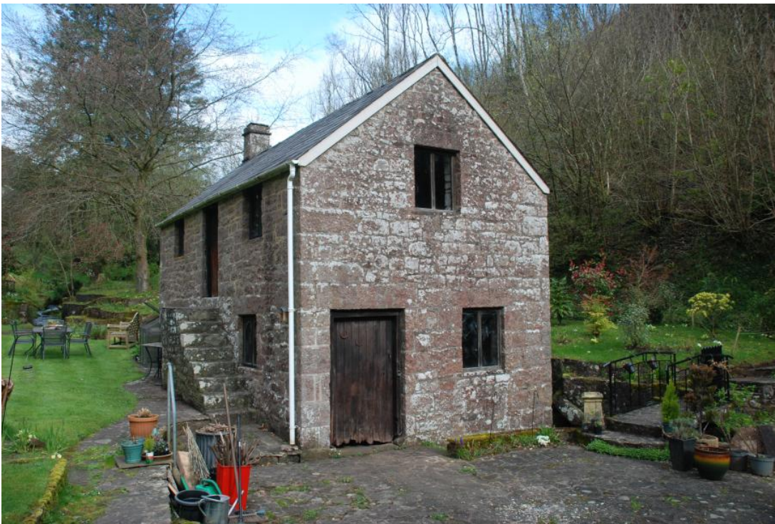
Plate 8: Cider Mill from south east with footbridge to right hand side.
