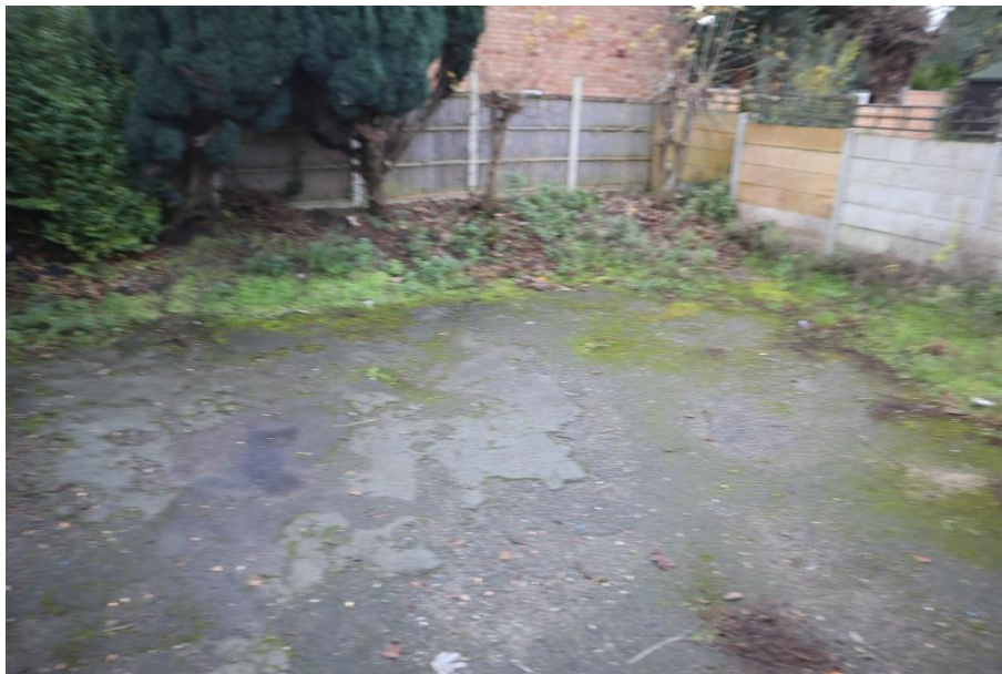
Figure 4.8. Yard to the south of the building
