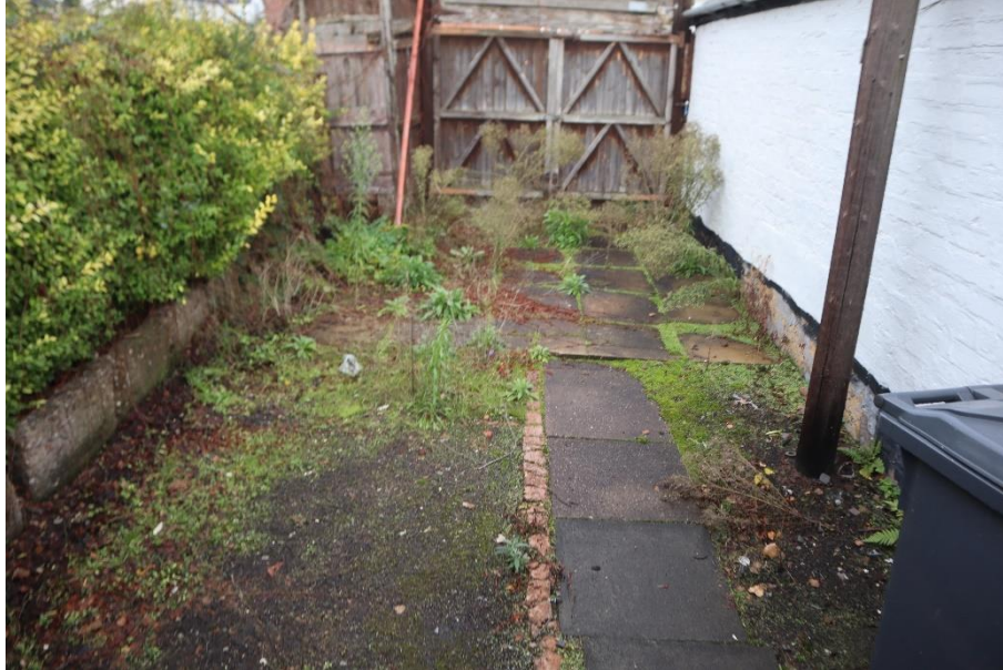
Figure 4.7. Yard to the west of the building
