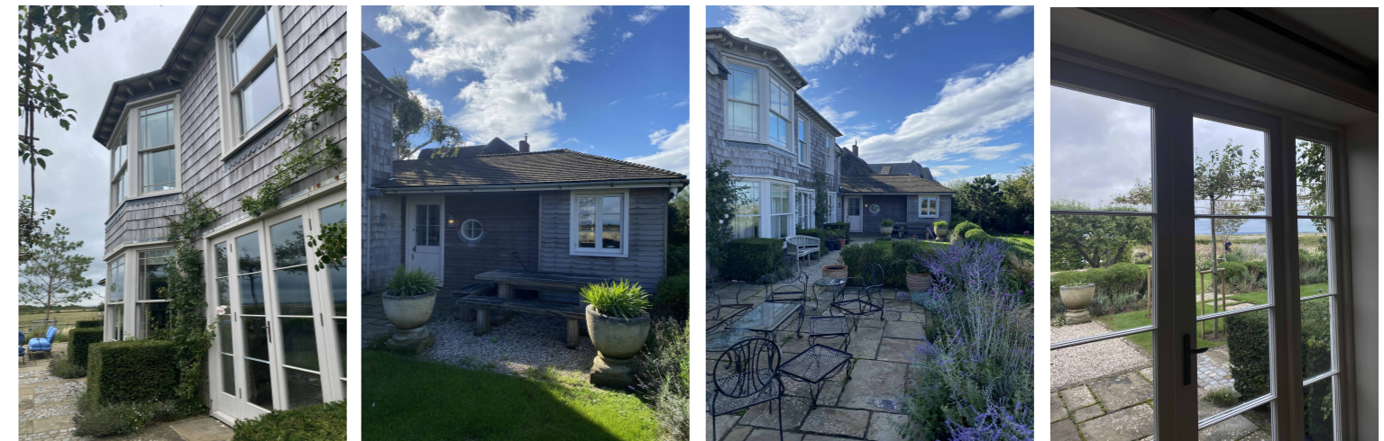
01 View of existing bay windows
