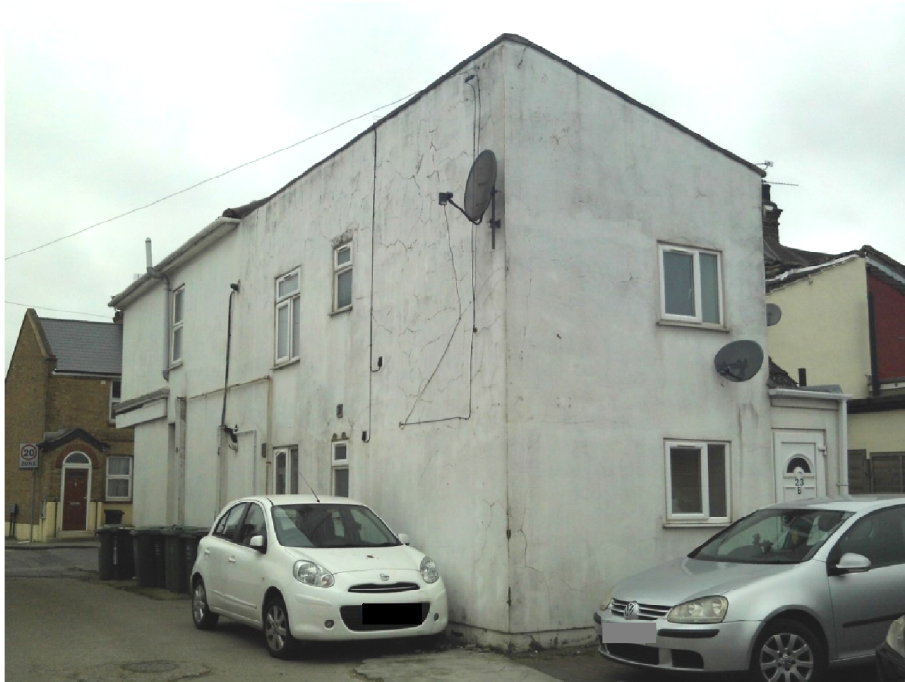
Looking west at the existing building from the access drive.
